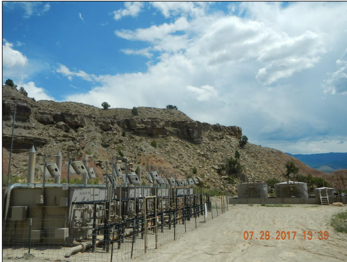
Separators and tank battery
