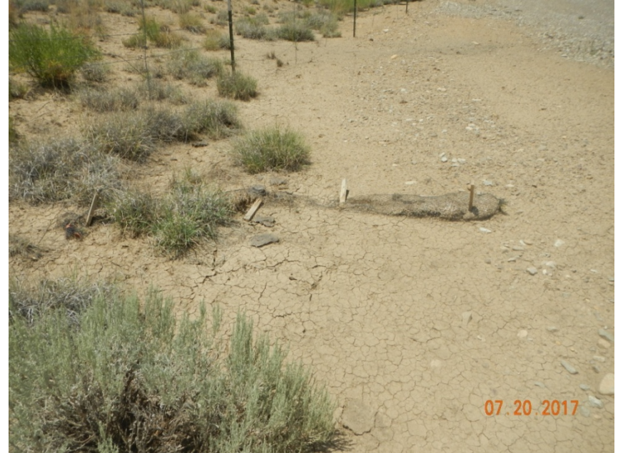
Photo 4: View of wattle full of sediment.
