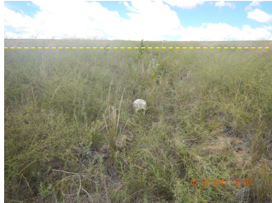
Photo 4: Photo taken from the west end of the location, facing west. Photo shows access road leading to the well has not been re-contoured. Yellow line indicates elevation of the adjacent reference area, hat in photo for reference to show depth of road.
