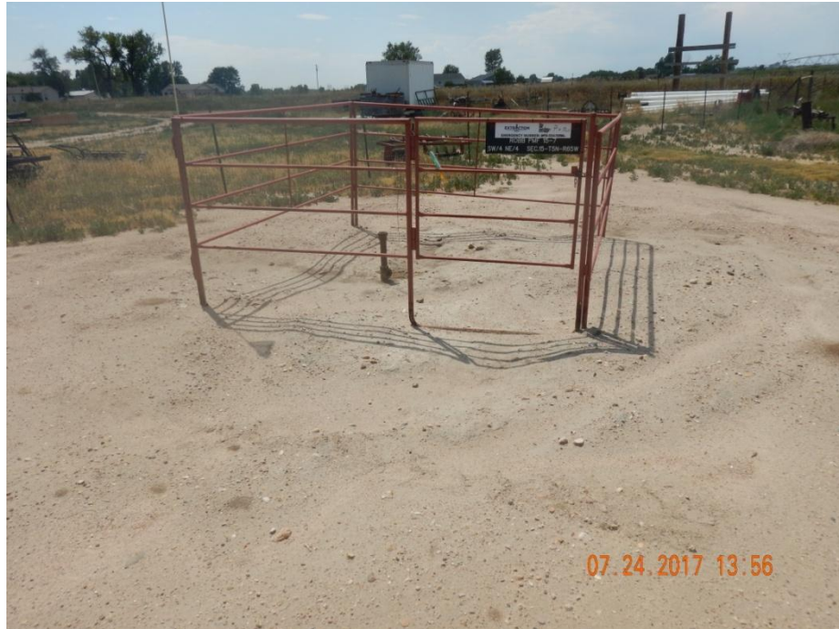
Photo 1: Photo taken from the Robb-PM #15-7 well location, facing west. Photo shows riser remaining at well location. Records indicate Bayswater as the last operator on record, however and extraction sticker has been placed on the sign.
