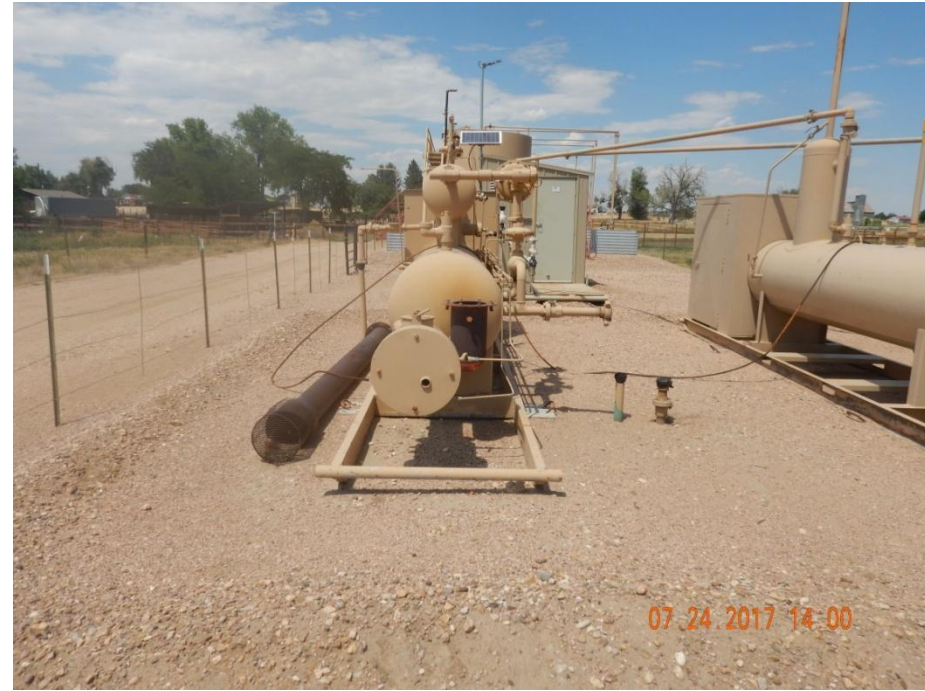
Photo 4: Photo taken from the Extraction battery location. Photo shows equipment associated with the Robb-PM F #15-7 appears to have been disconnected, but has not been removed per 1004.a. Photo also shows risers that have not been marked or removed per phase I and II of the May 2, 2017 Flowline or Pipeline NTO, and per rule 1004.a.
