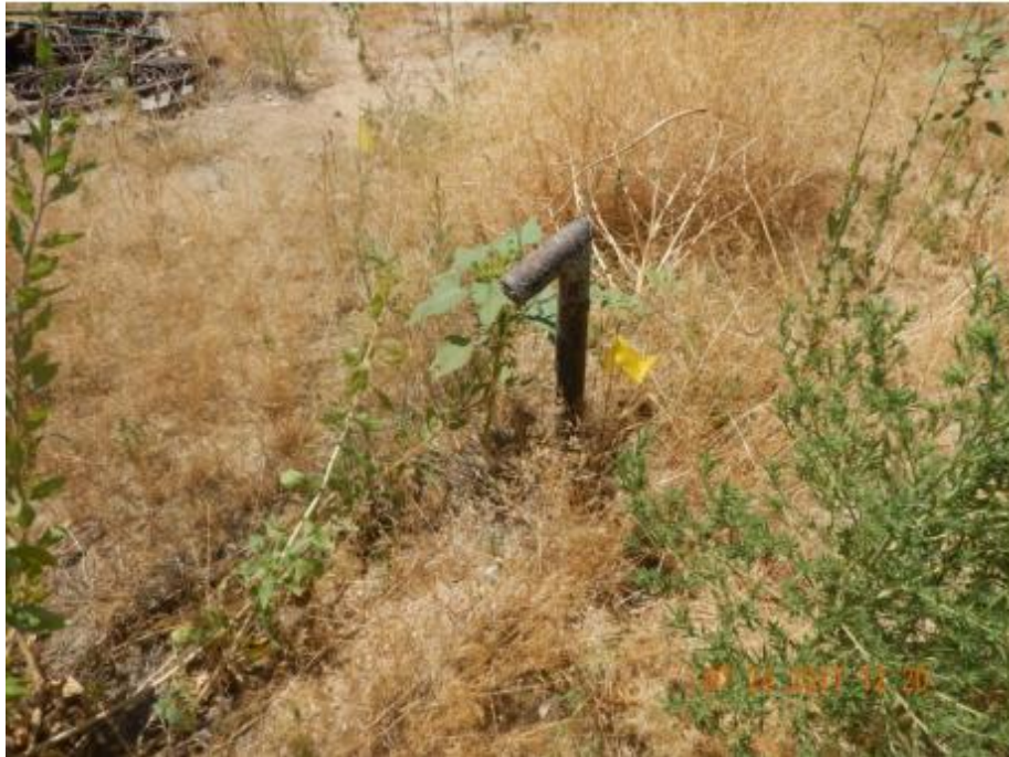
Photo 3: Photo taken west of the well. Photo shows vent pipe from line. If line from well to former battery has been abandoned, this should be removed.
