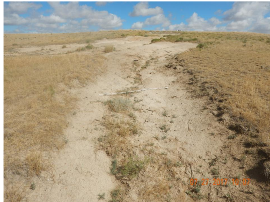
Photo 6: Photo taken from the southeast end of the unvegetated area, facing north. Photo shows large un-vegetated area experiencing erosion. Photo shows stormwater and sediment control BMPs have not been installed per CAs from inspection doc. # 682501478 and doc # 682501125. Areas have continued to degrade due to erosion. 6 foot measuring stick for reference.
