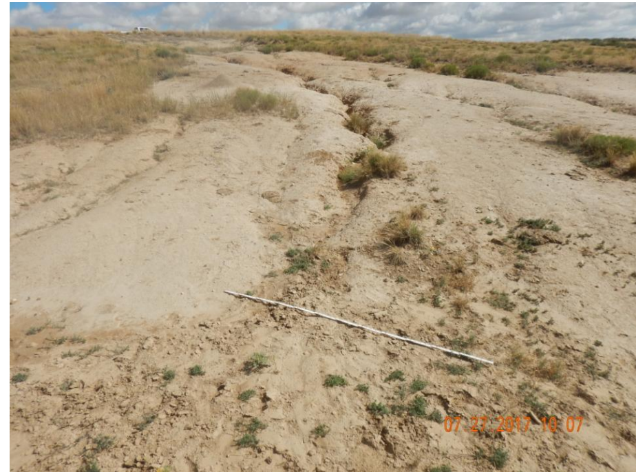
Photo 4: Photo taken from the southwest end of the unvegetated area, facing north. Photo shows large un-vegetated area experiencing erosion. Photo shows stormwater and sediment control BMPs have not been installed per CAs from inspection doc. # 682501478 and doc # 682501125. Areas have continued to degrade due to erosion. 6 foot measuring stick for reference.
