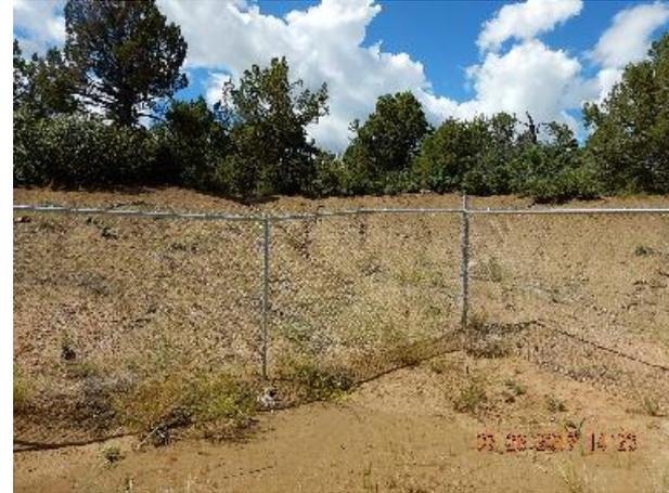
**Photo 6: Erosion channels and rilling in NE corner of cut slope carrying sediment onto location.**
