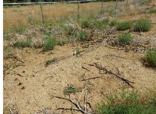
**Photo 4: Waddles with backside full of sediment.**
