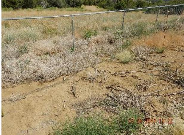
**Photo 5: Waddles with backside full of sediment.**
