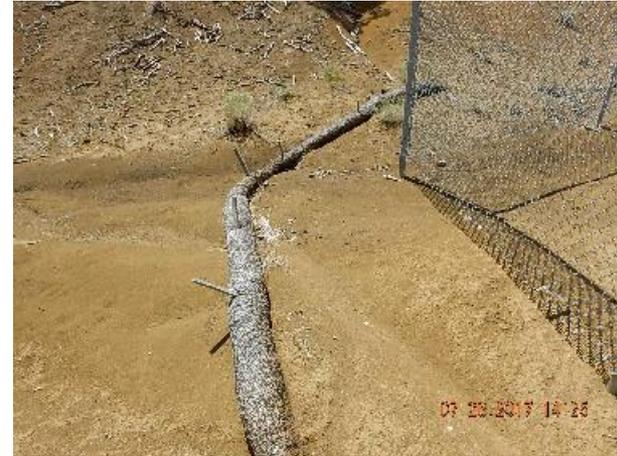
**Photo 8: Waddle and sediment flow in SW corner.**
