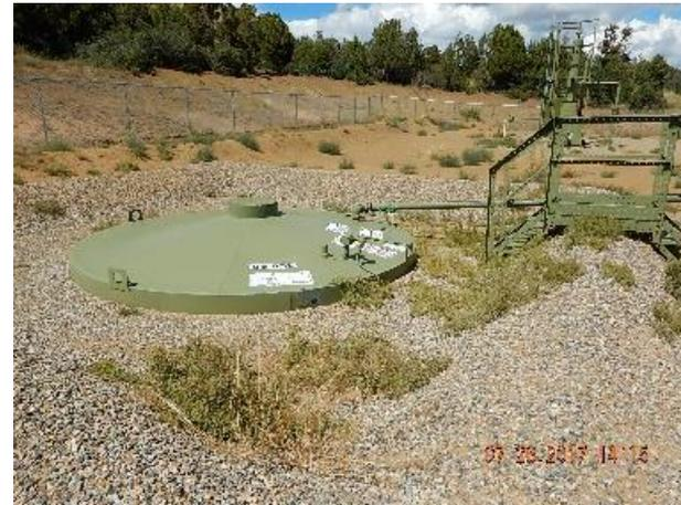
Photo 2: Weeds on berms and base of containment.
