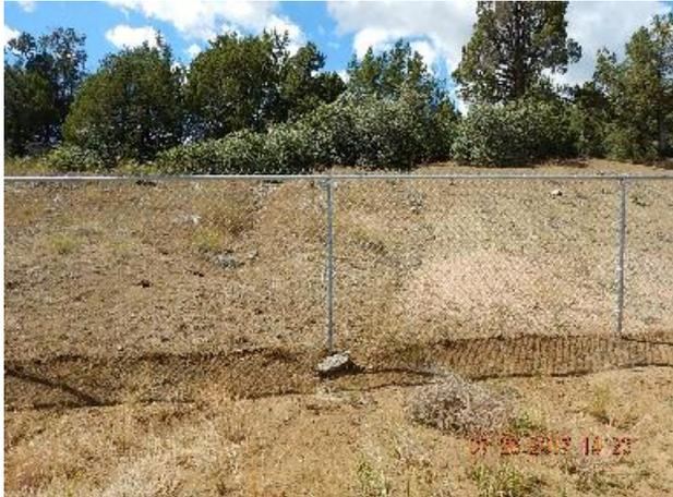
**Photo 7: Erosion around fence post concrete.**
