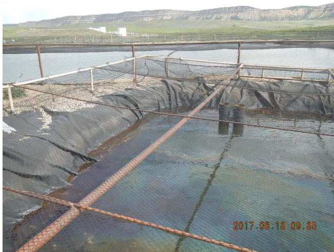
Pit with hydrocarbon sheen.
