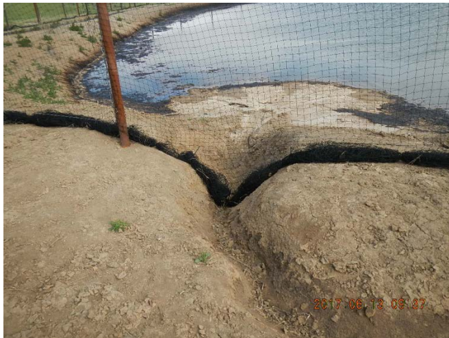
Pit Facility ID 116589 with sediment flow into pit.
