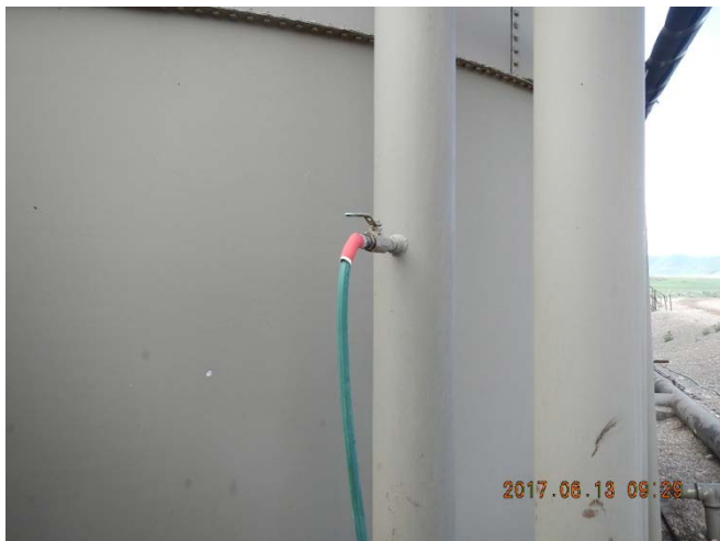
Fluid being discharged to trough via garden hose from Tank #5. App 15 gpm.
