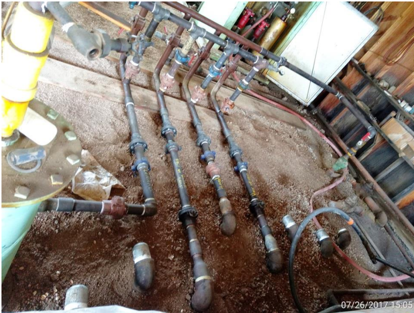
Inside separator housing Note: unidentified risers (5) 39.979830, -104.944194
