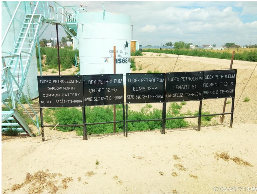
Battery Signage Corrective action: Emergency contact info missing
