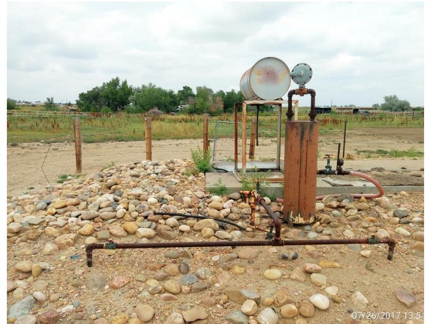
Supply scrubber, note: unidentified 1" poly riser 39.983924, -104.947282
