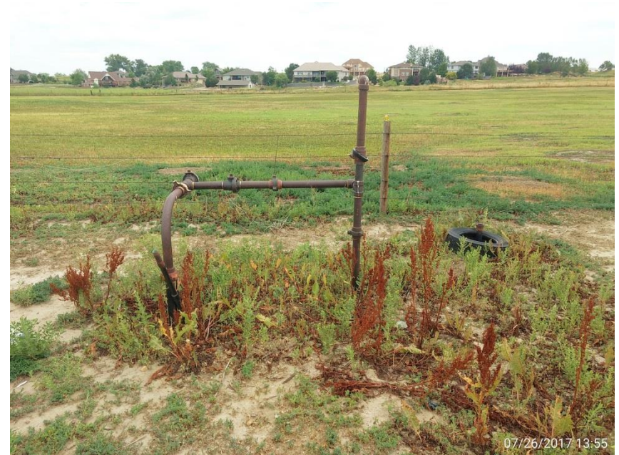
Unidentified risers both 2" steel, and 1" poly. 39.983979, -104.946858
