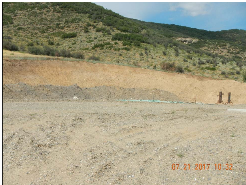
Photo 3. Cuttings and drilling equipment stored on location.
