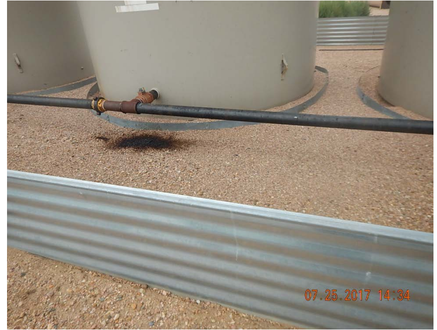
Photo 4: Stained soil at loadout
