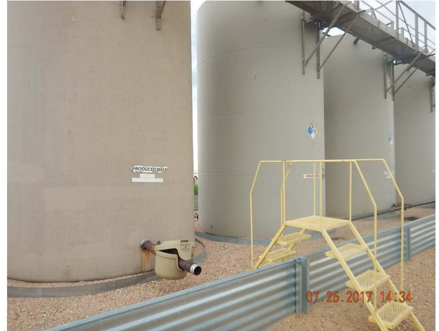
Photo 5: No capacities on production tanks. No safety placarding on produced water tank.
