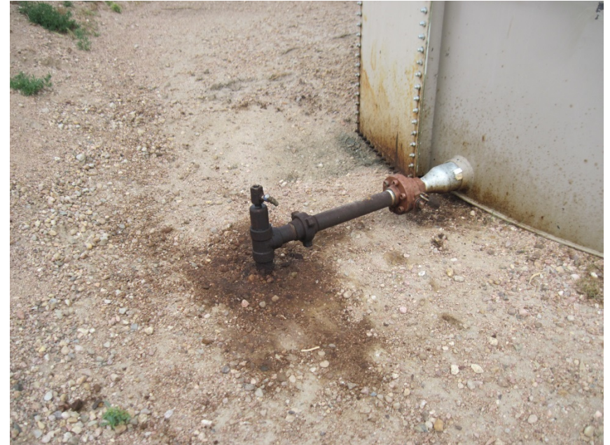
Stained soil at drain line on tank
