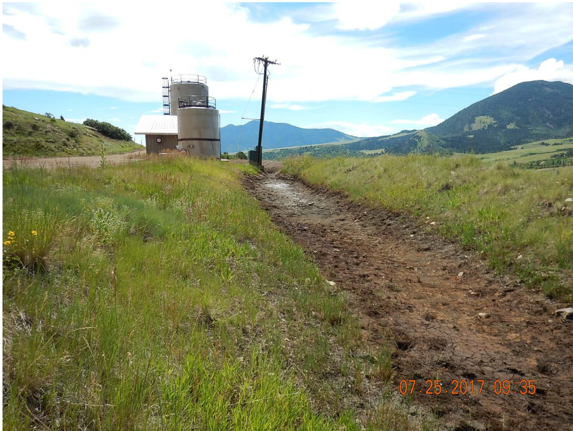
Stained soil in containment. Calculation of area indicate that spill is less than 5 bbl and not reportable under Rule 906.
