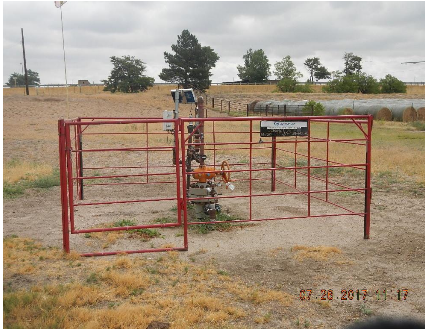
Photo 1 Wellhead from west
