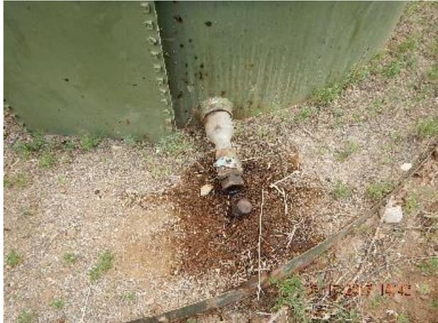
**Photo 3: Leaking production tank valve.**
