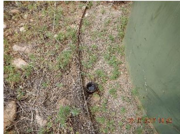
Photo 2: 3" riser beside tank with no plug and stained soil around it.
