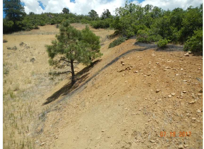
Photo 2: View of the southern portion of the project area from the southwestern corner facing eastward. Black netting debris needs to be properly installed or removed.
