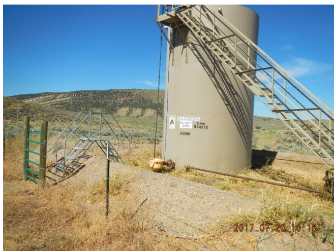
Tank battery bermed.
