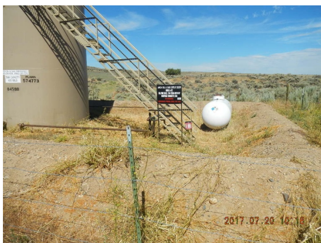
Tank battery bermed.
