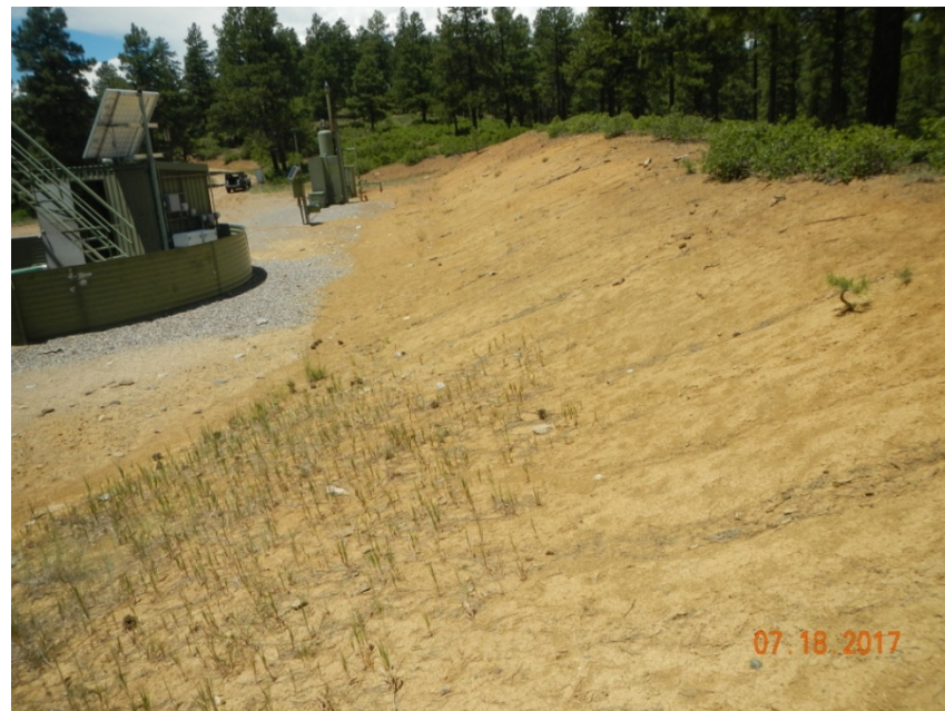
Photo 2: View of the northern portion of the project area from the northeastern corner facing westward. Revegetation on the northern cut-slope is sparse.
