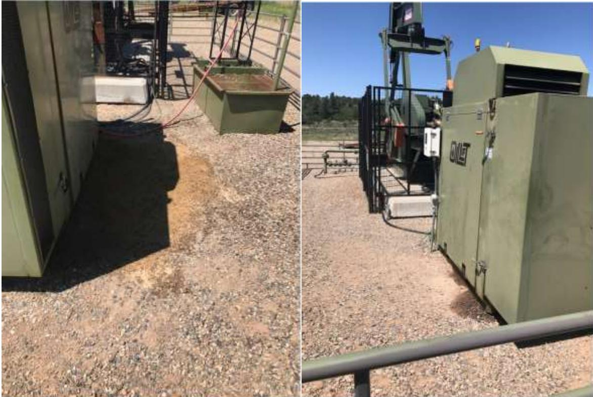
Photos of stained areas after crew shoveled up all stained soils into bags to be taken to soil box at Durango Operations Center for remediation at IEI. No manifest available as soil box is for all soils cleaned up which are at a non-reportable amount. As demonstrated in photos below the stained soils were removed from around equipment, bagged for deposit into BP soil box and clean soil was placed into the remediated area. All stained soils have been cleaned up closing out CA in COGCC inspection.
