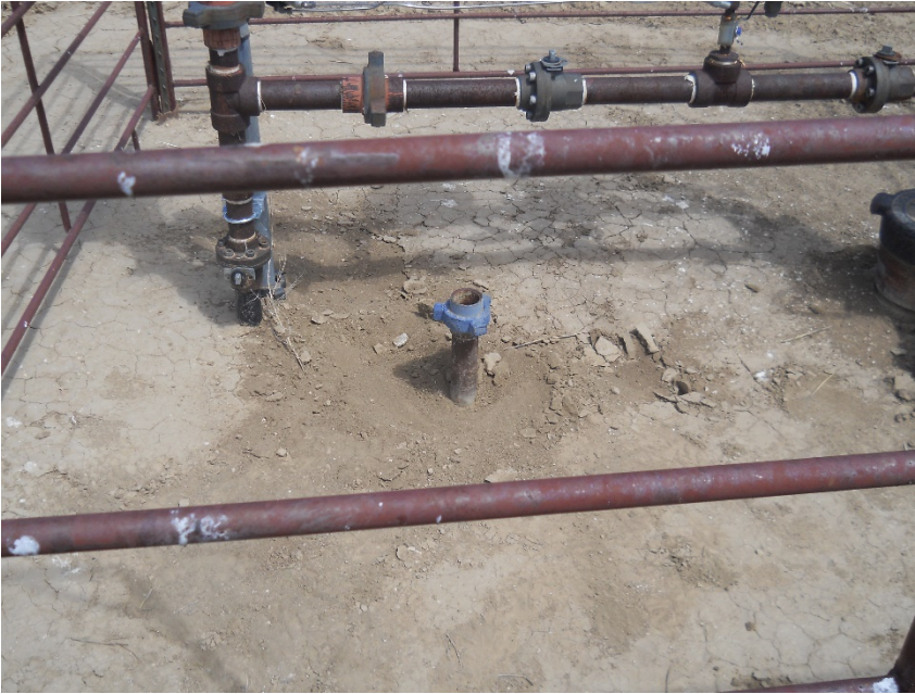
3) Wellhead looking north with unused riser
