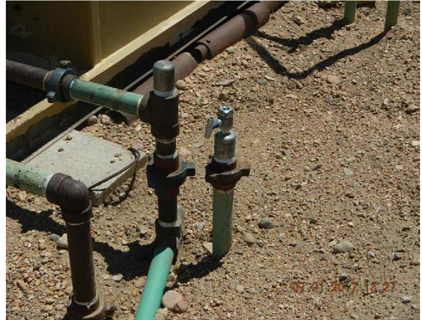
2" unmarked riser at separator
