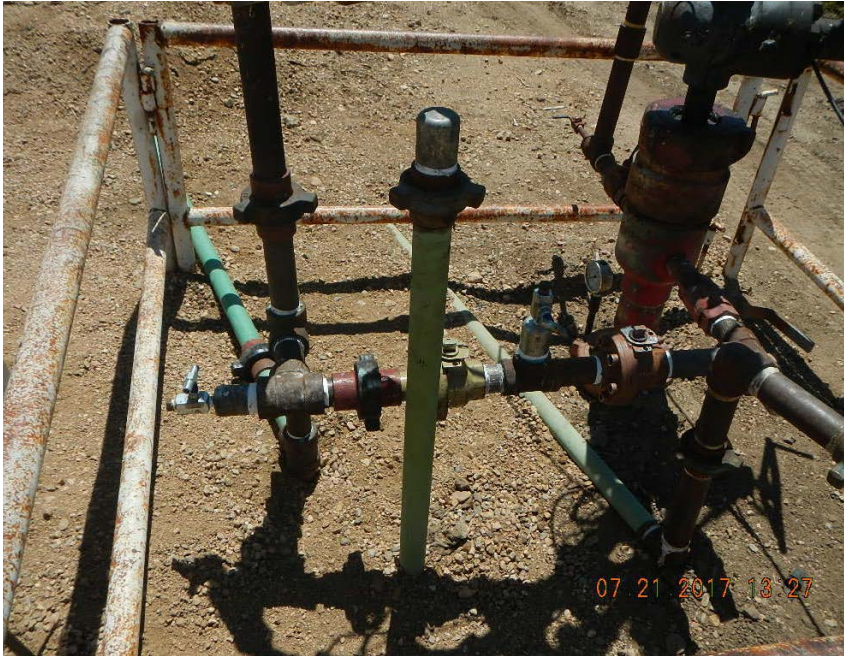
2" unmarked riser at wellhead
