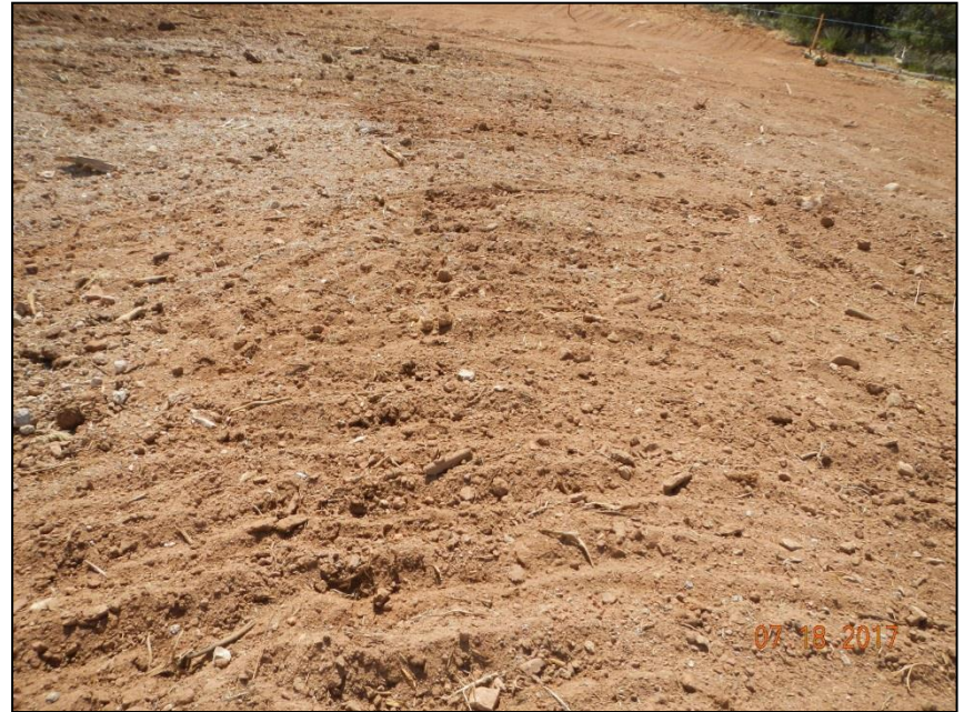
Photo 11. Newly disturbed area, seeding/stabilization not yet performed
