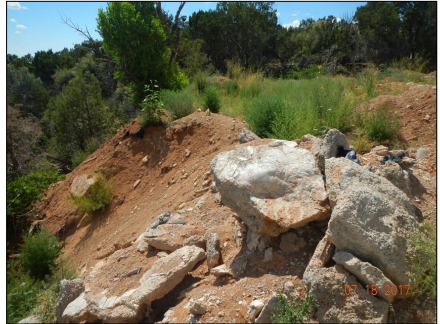
Photo 4. Spoil piles eroding into drainage, no stormwater/sediment controls
