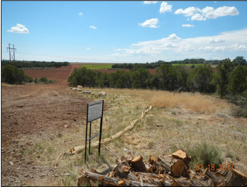
Photo 10. Newly disturbed area NW corner of location, well sign, slash pile. Note perimeter wattles have not been re-installed
