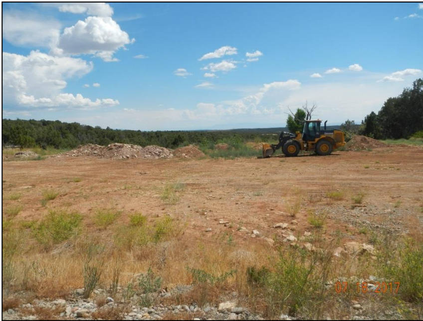
Photo 5. Widened area where drainage has been filled in by dumping spoil and waste materials from unknown origin
