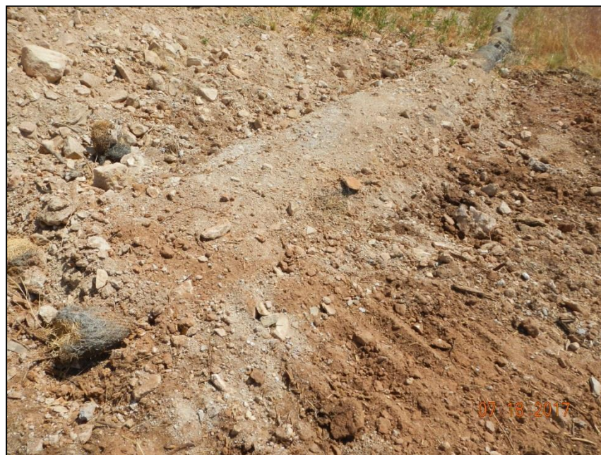
Photo 13. Straw wattle covered in material and in disrepair NW corner
