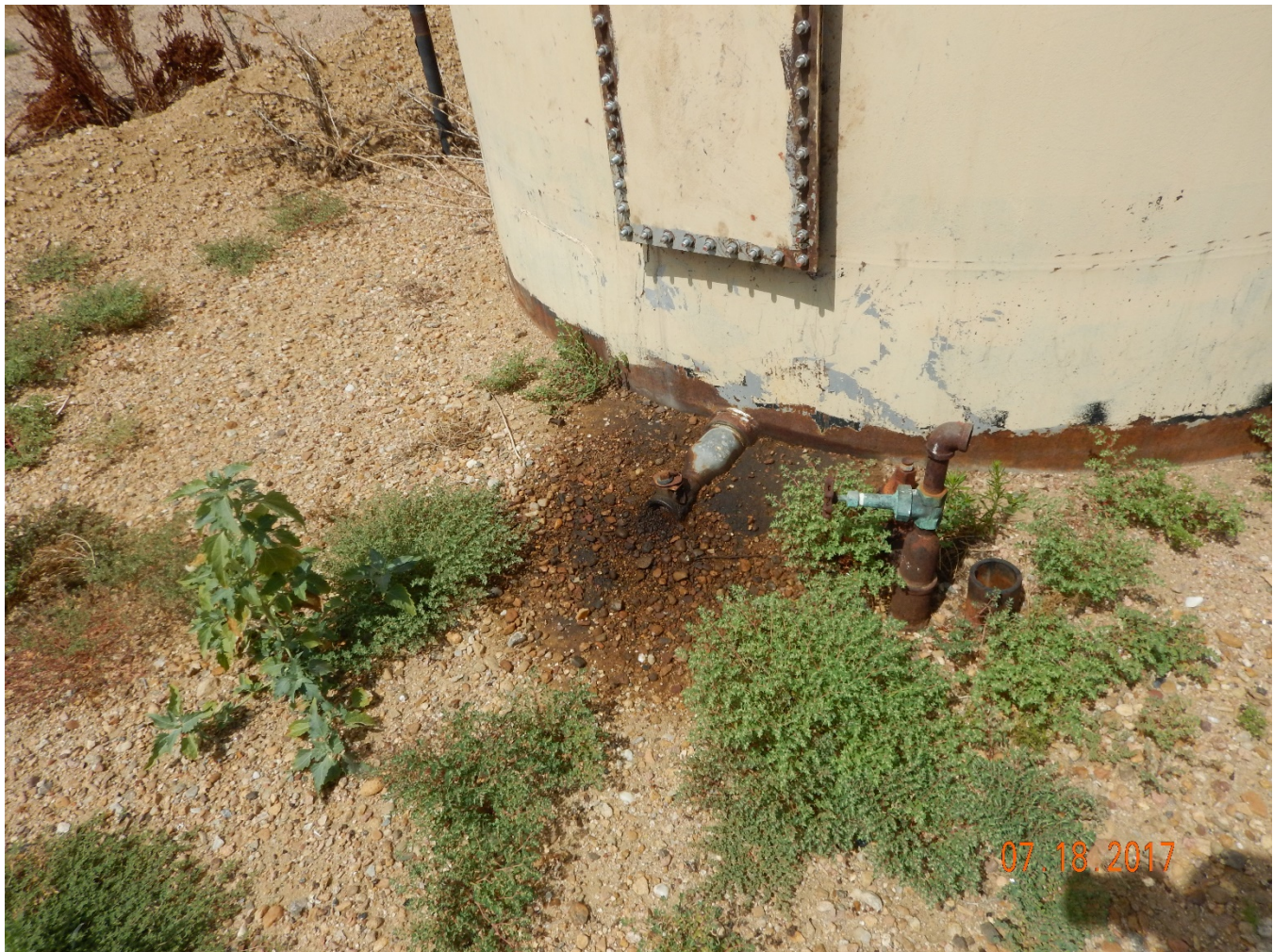
Figure 4 - Localized, oil-stained soil at south tank.
