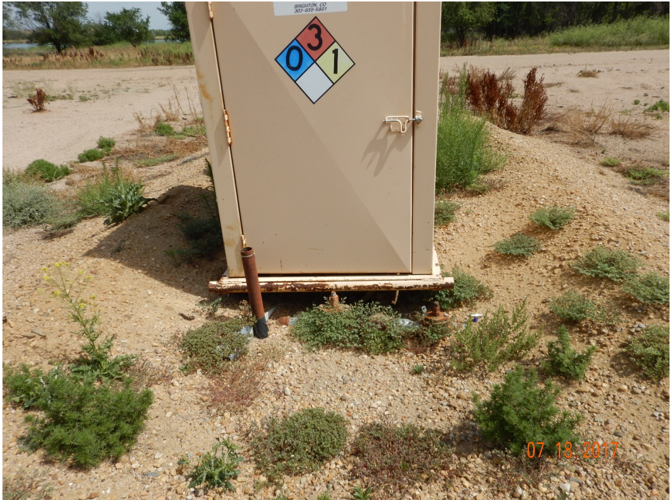
Figure 5 - Uncapped, unmarked flowline riser at SW corner of separator.
