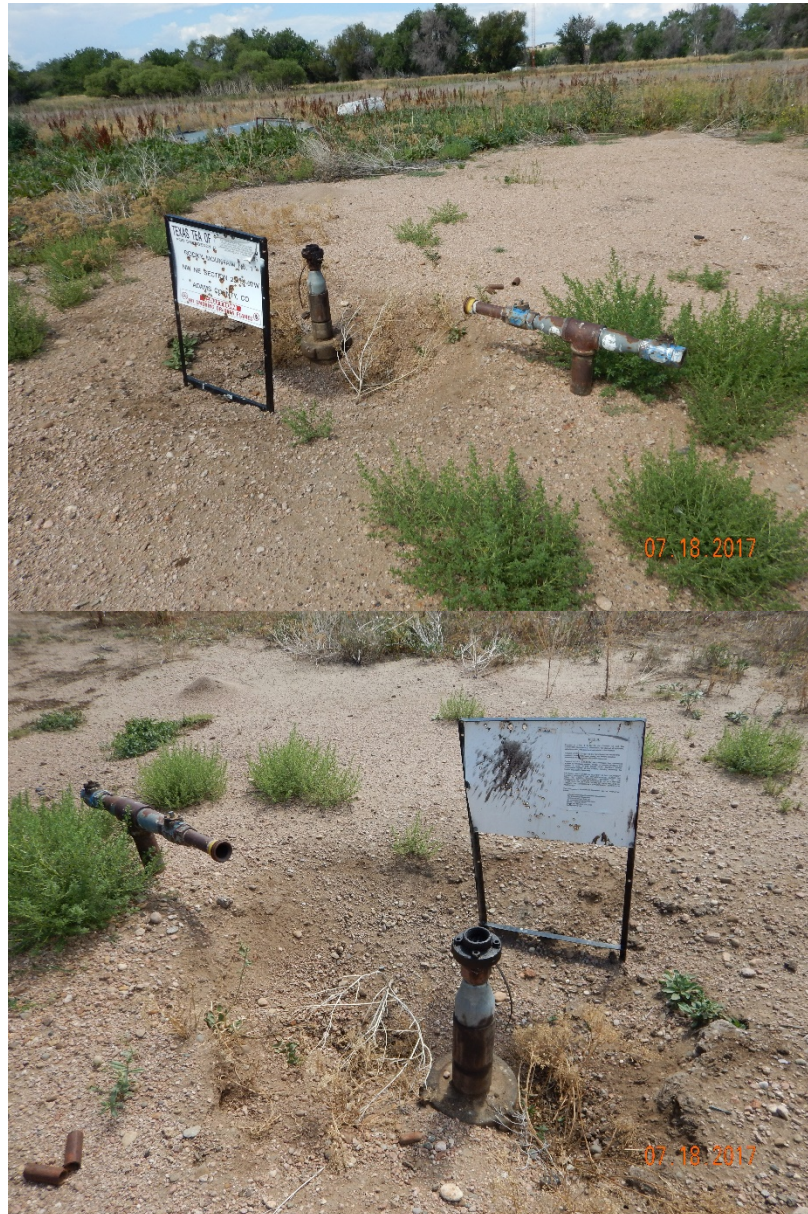
Figure 1 - Rocky Mountain II 1 wellhead sign, wellhead, and flowline riser. Note: flowline riser is neither capped, painted, nor tagged (as required by 2017 Flowline NTO). Both wellhead and flowline are open to atmosphere and wellhead is sitting in a depression.
