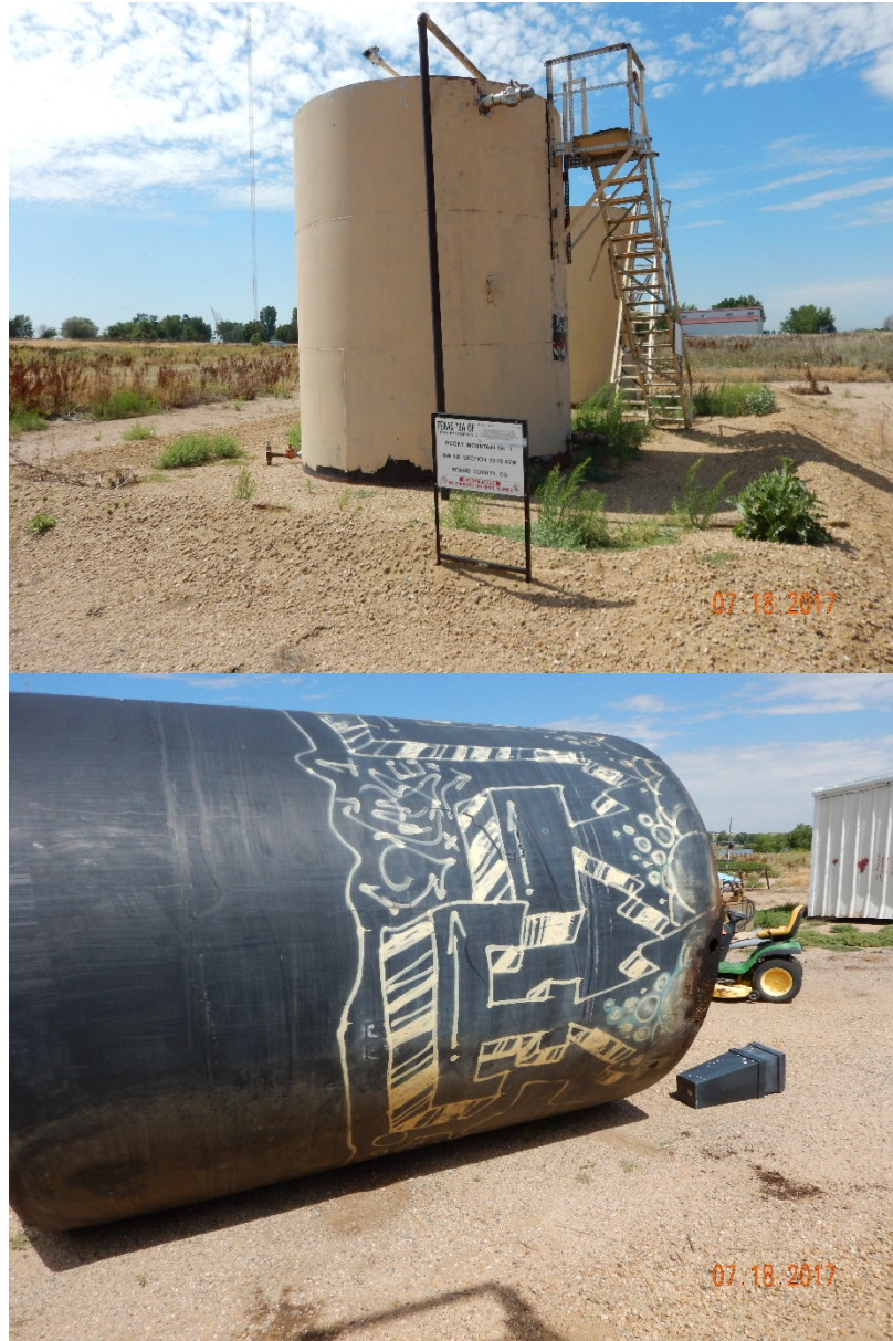
Figure 3 - Tank battery (top) with unused, overturned tank outside of berm (bottom).
