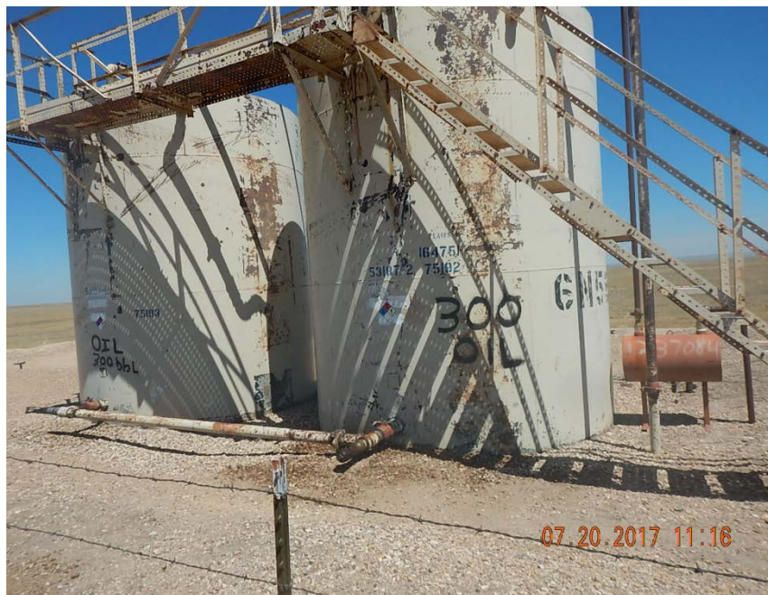
Photo 1: Tanks are rusted
