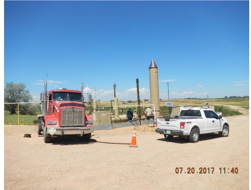
Photo 4 Separators from east
