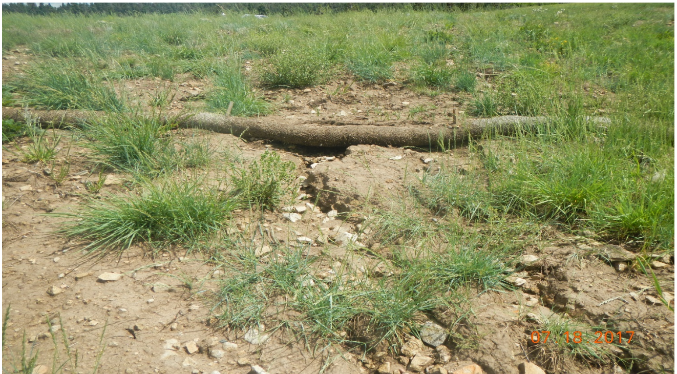
photo 6: Stormwater is flowing underneath the wattle causing erosion.
