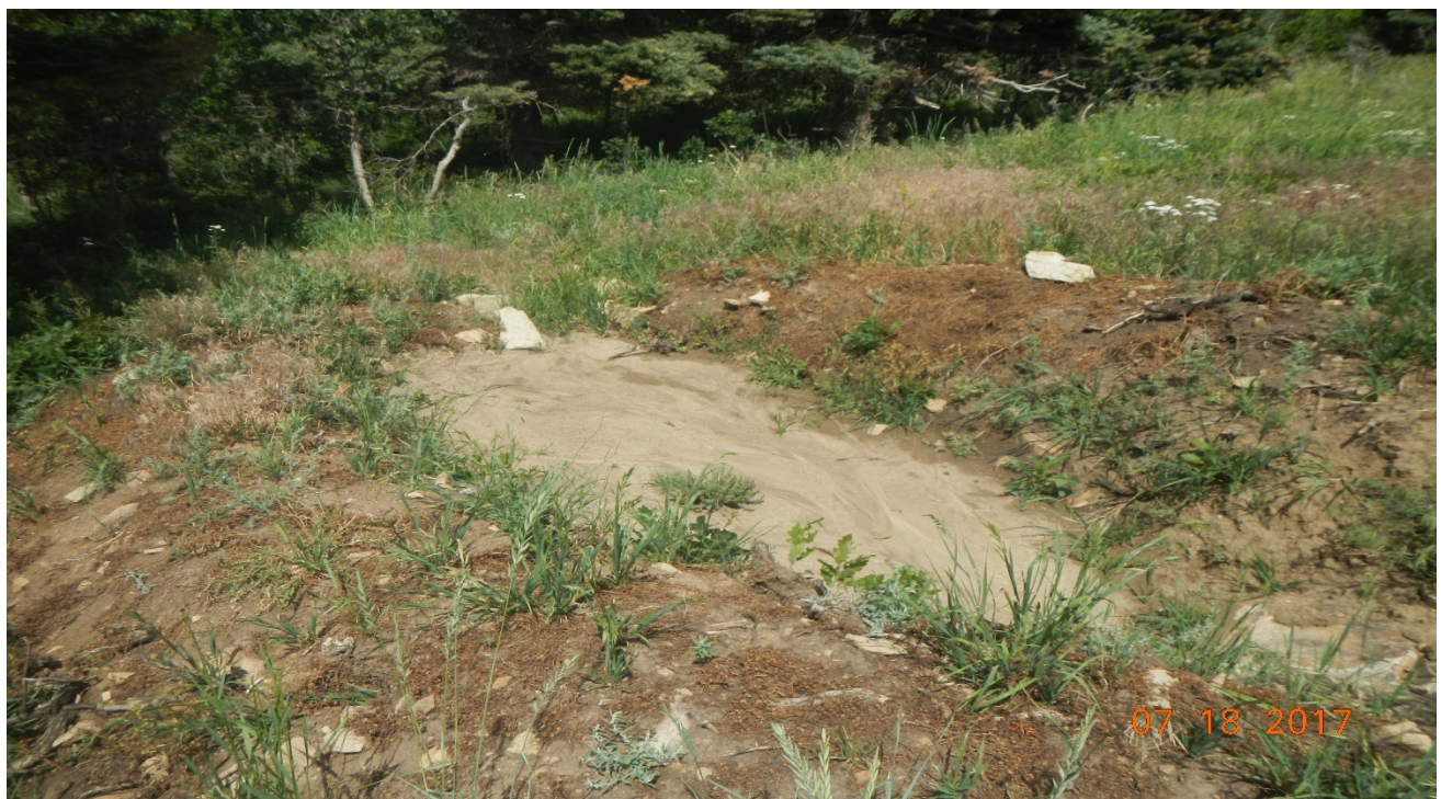
photo 2: The sediment trap has filled in with sediment and needs to be maintained.
