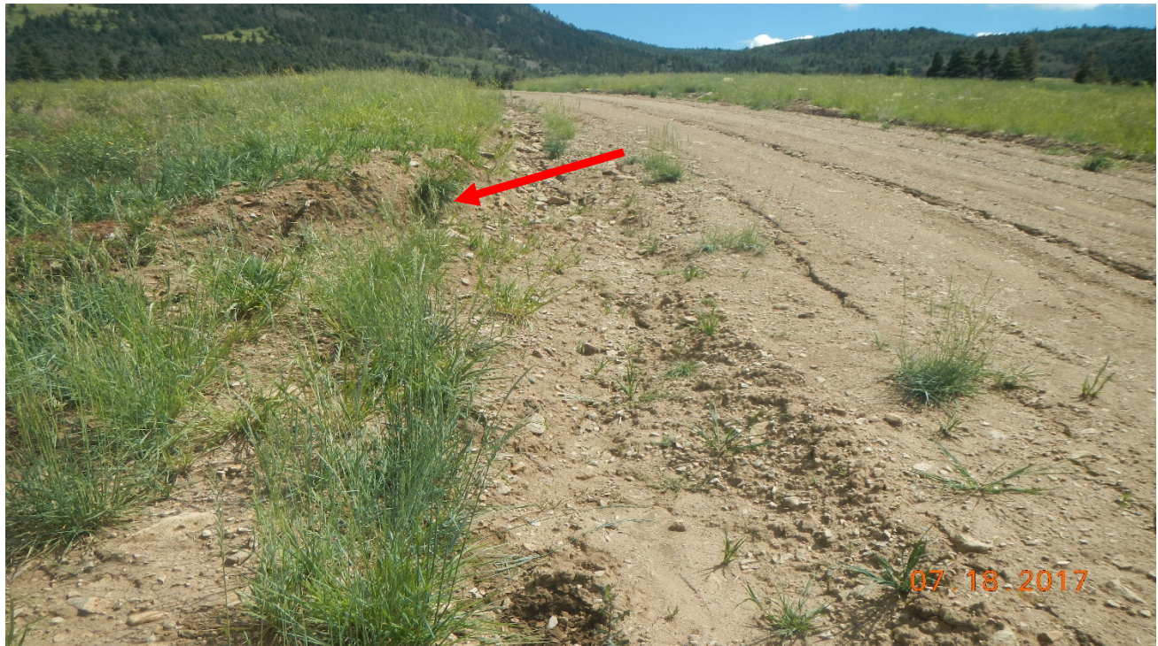
photo 1: Facing south along the access road toward the location. Stormwater is not adequately directed toward the sediment trap shown in photo below.
