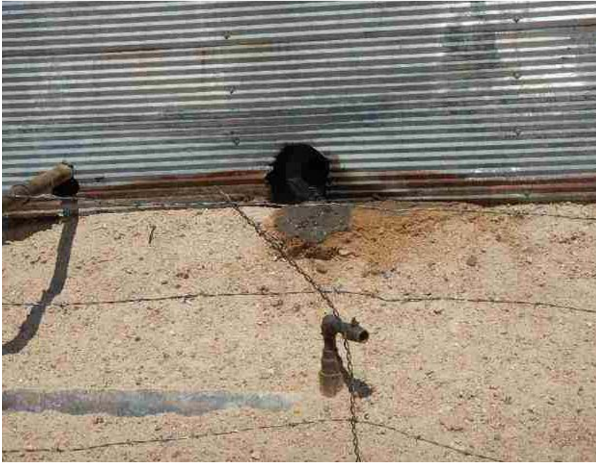
Photo from prior inspection for comparison
