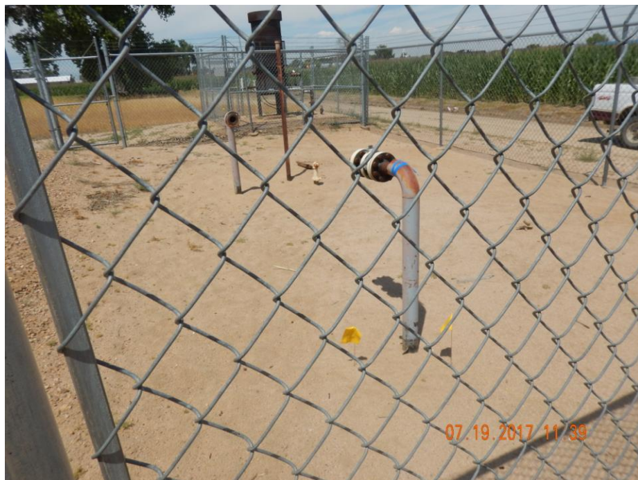
Photo 3: Photo taken from the battery location. Photo shows four (4) risers that appear to be abandoned.
