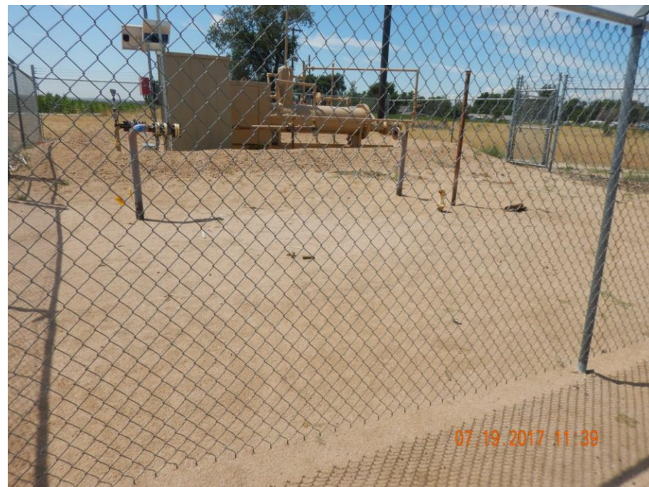
Photo 4: Photo taken from the battery location. Photo shows four (4) risers that appear to be abandoned.
