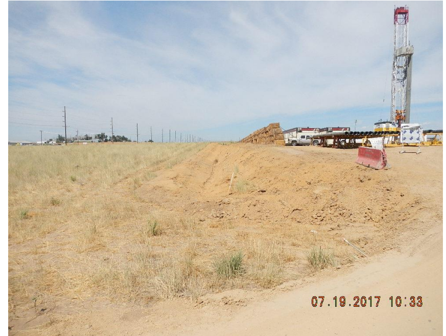
Photo 2 Ditch and hydro mulch at entrance from east
