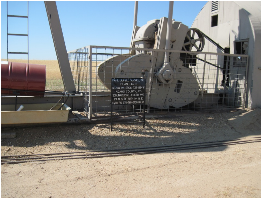
wellhead, pump jack, sucker rods and clean up pump jack
