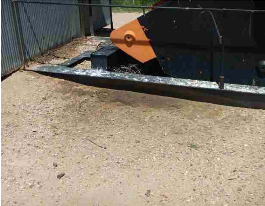
Photo from prior inspection for comparison
