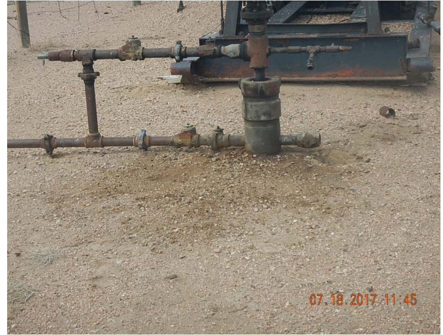
Photo 1: Stained soil at wellhead, no bradenhead at surface
