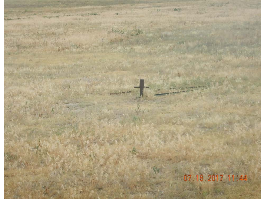
Photo 3: Deadman markings in disrepair
