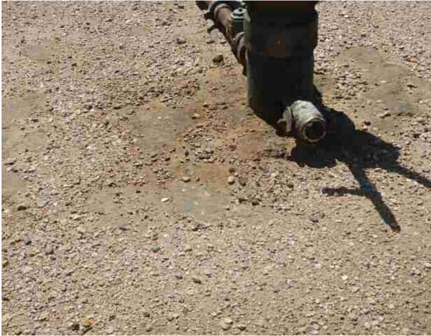
Photo from prior inspection for comparison
