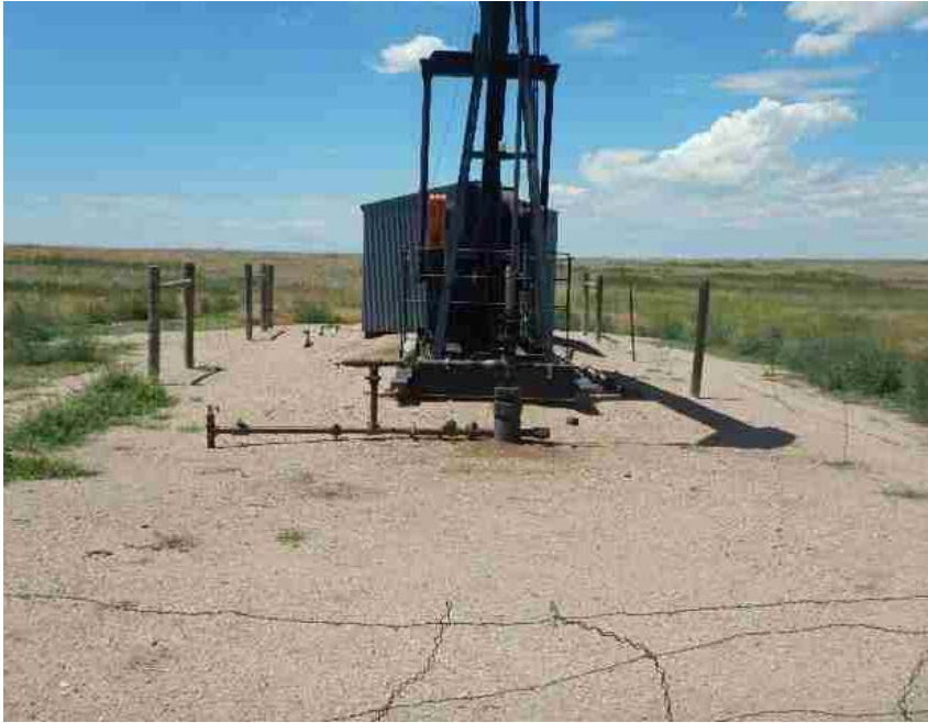
Photo from prior inspection for comparison
