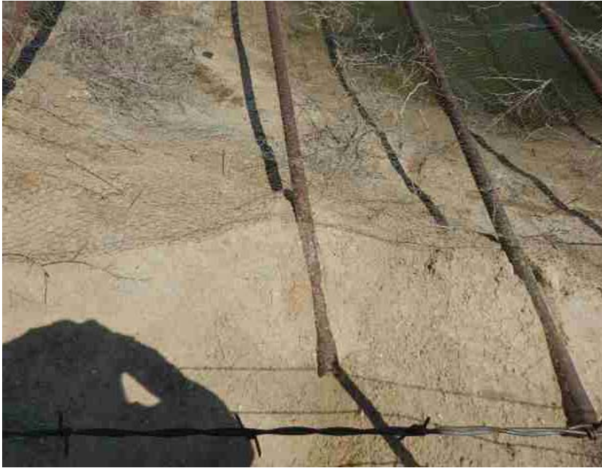
Photo from prior inspection for comparison
