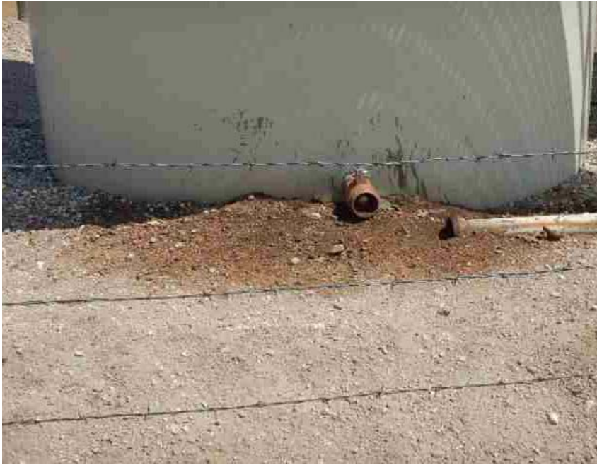
Photo from prior inspection for comparison
