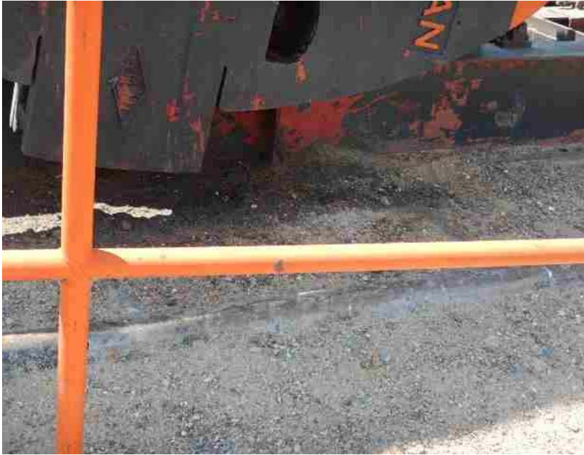
Photo from prior inspection for comparison
