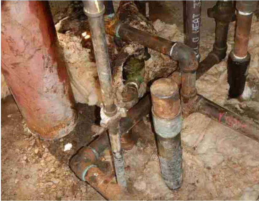
Photo from prior inspection for comparison
