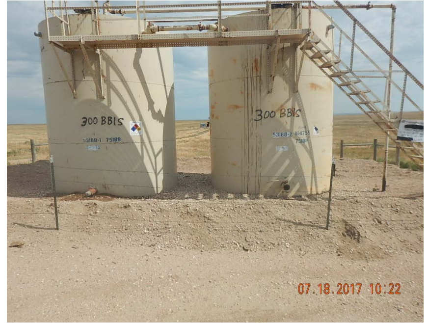
Photo 6: Damaged placard on east tank, tanks are placarded
