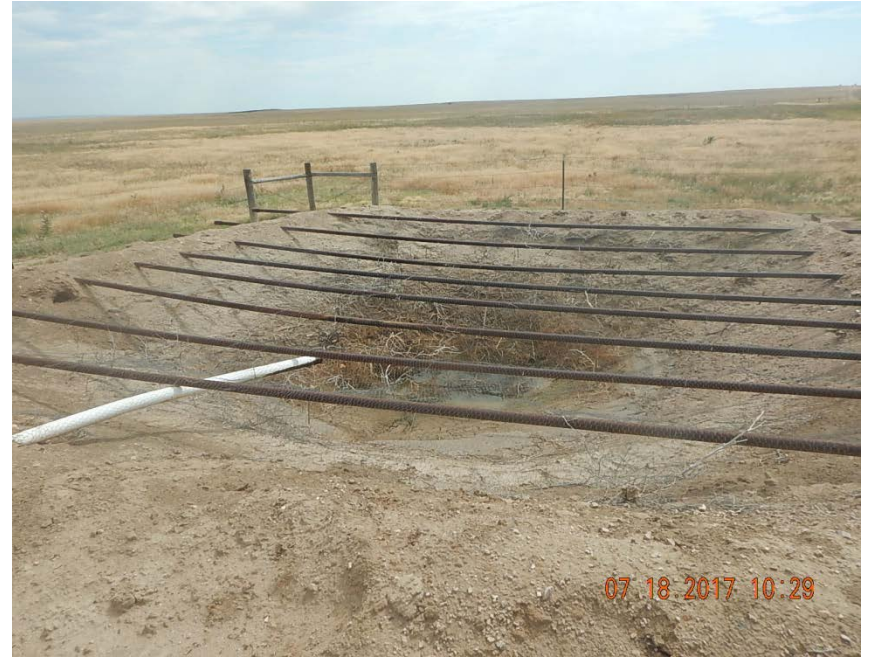
Photo 7: Mesh repaired
