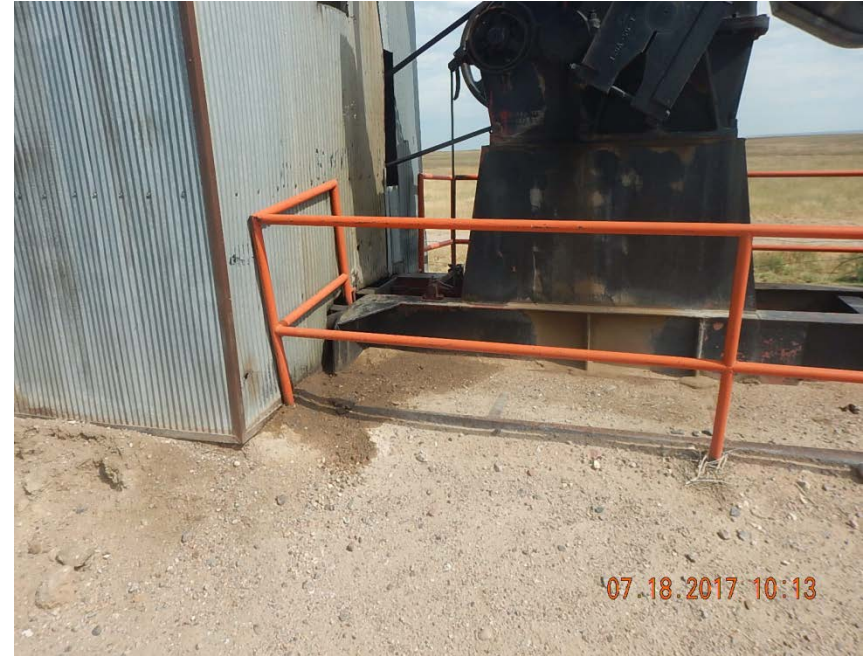
Photo 3: Stained soil at pump jack and engine
