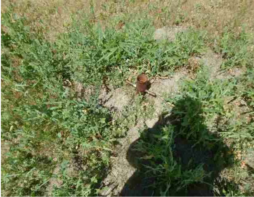
Photo from prior inspection for comparison
