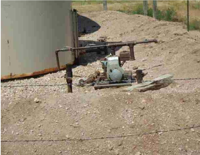
Photo from prior inspection for comparison
