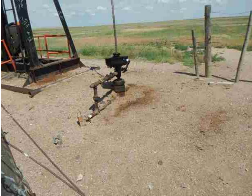
Photo from prior inspection for comparison
