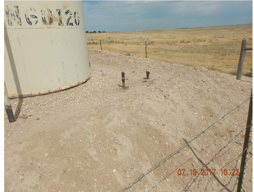
Photo 5: Unused pump removed. Two unused risers.
