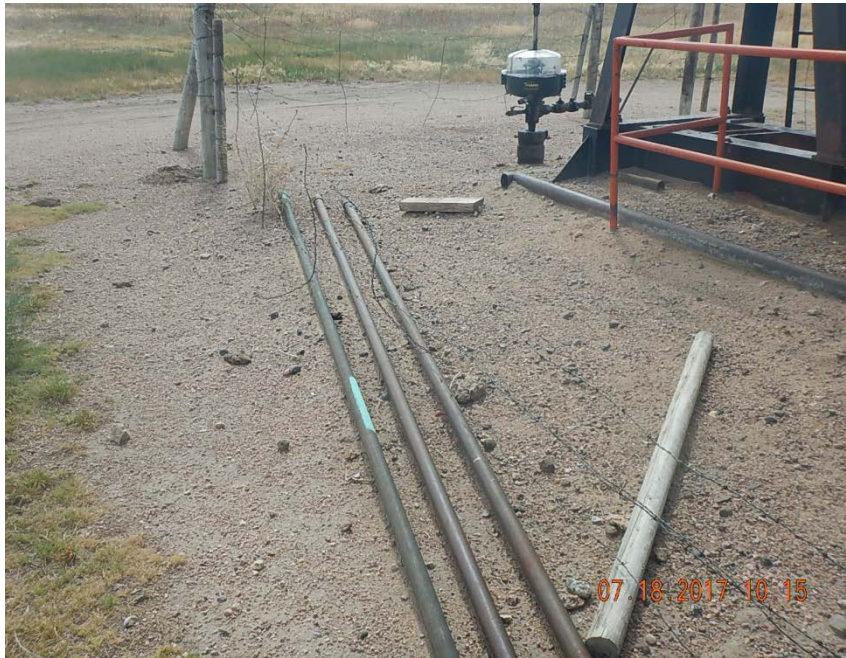
Photo 14: Unused equipment at pump jack.
