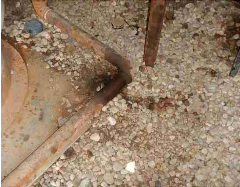
Photo from prior inspection for comparison
