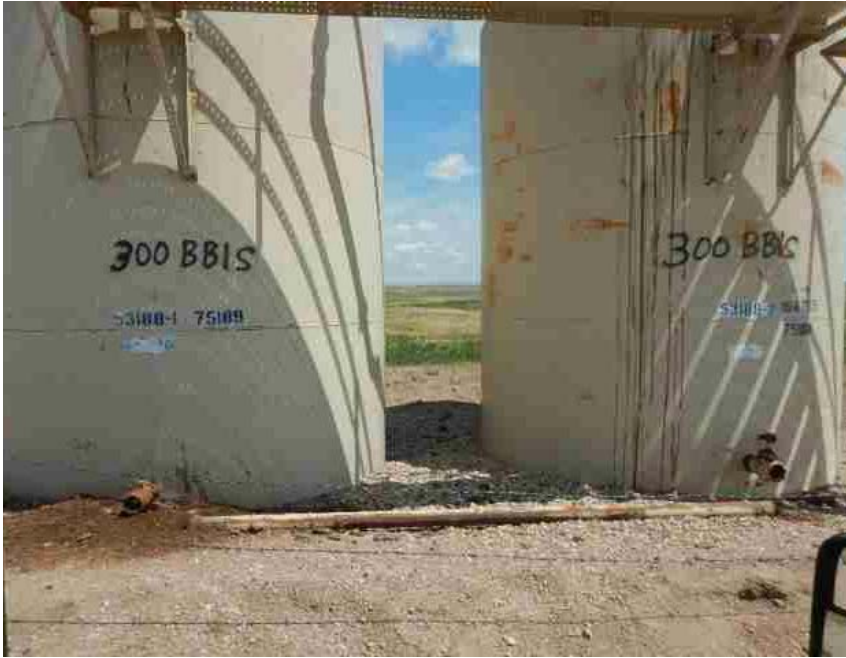
Photo from prior inspection for comparison
