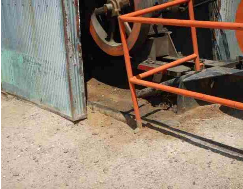
Photo from prior inspection for comparison
