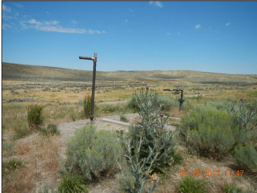
Photo 2. Unused 2" steel riser on left, unused 3" steel riser on right. Noxious weeds in foreground.
