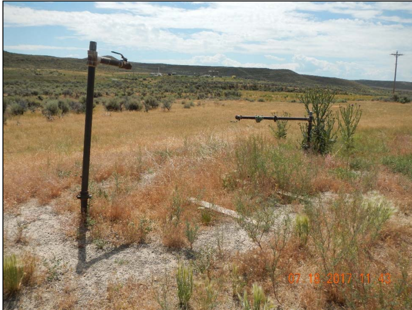
Photo 2. Unused 2" steel riser on left, unused 3" steel riser on right. Noxious weeds visible adjacent to 3" riser.
