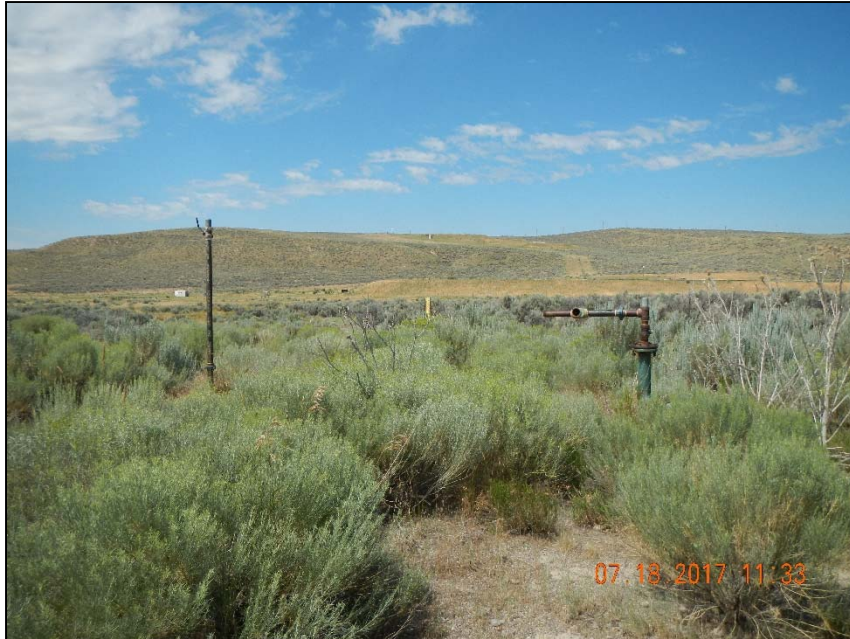
Photo 2. Unused 2" steel riser on left, unused 3" steel riser on right.
