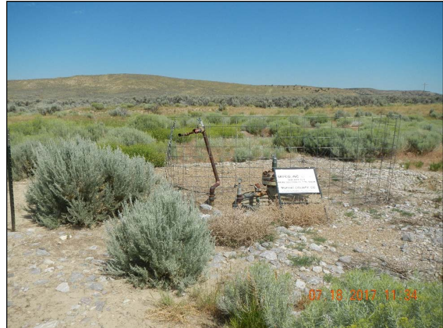
Photo 3. Unused 2" steel riser at wellhead.
