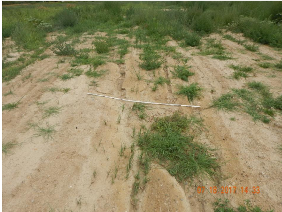
Photo 7: Photo taken from the north end of the location. Photo shows stormwater erosion occurring throughout the reclamation / remediation area. 6 foot measuring stick for reference. Location appears to have had a seeding attempted, however location was not seeding along the contour of the slope. This has facilitated erosion on the location.
