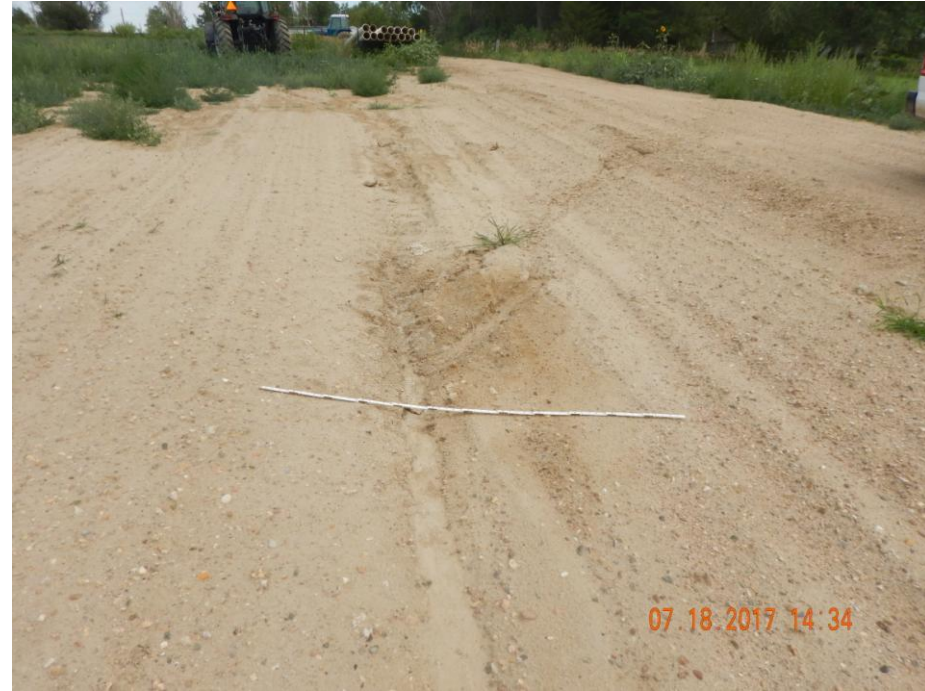
Photo 8: Photo taken from the north end of the location. Photo shows stormwater erosion occurring throughout the reclamation / remediation area. 6 foot measuring stick for reference. Location appears to have had a seeding attempted, however location was not seeding along the contour of the slope. This has facilitated erosion on the location.
