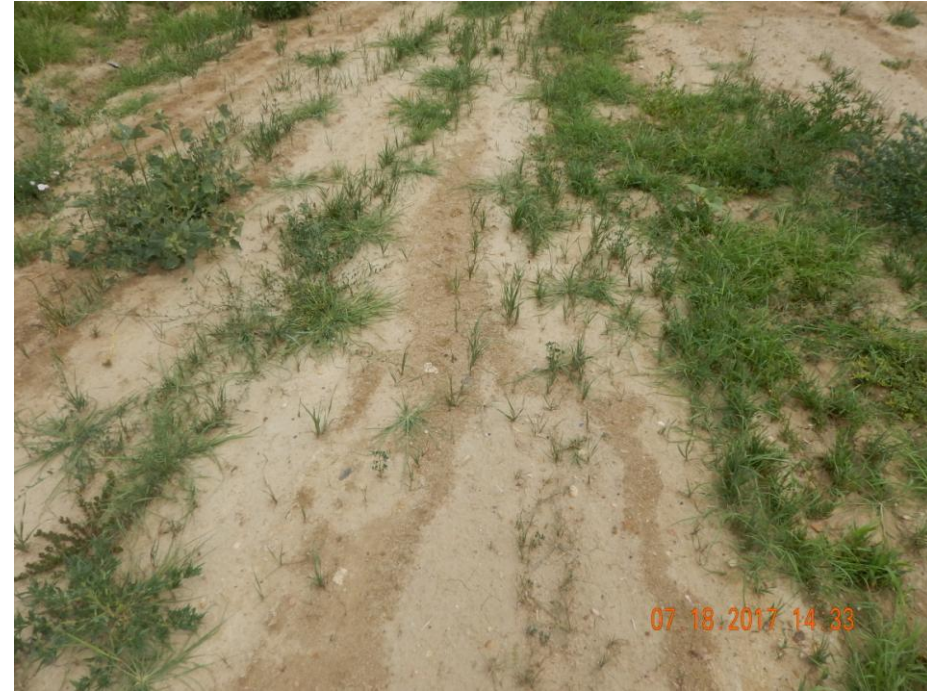
Photo 6: Photo taken from the north end of the location. Photo shows vegetative growth (likely) from a seeding. Appears location had been reseeded, however evidence of germination is scarce with the majority of the location predominantly exposed soil. Also, location was not seeding along the contour of the slope, which has facilitated erosion on the location.
