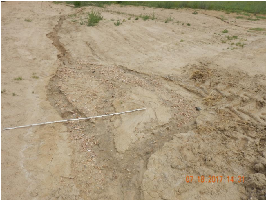
Photo 1: Photo taken from the southwest end of the location, facing southeast. Photo shows stormwater erosion occurring throughout the reclamation / remediation area. 6 foot measuring stick for reference. Location appears to have had a seeding attempted, however location was not seeding along the contour of the slope. This has facilitated erosion on the location.
