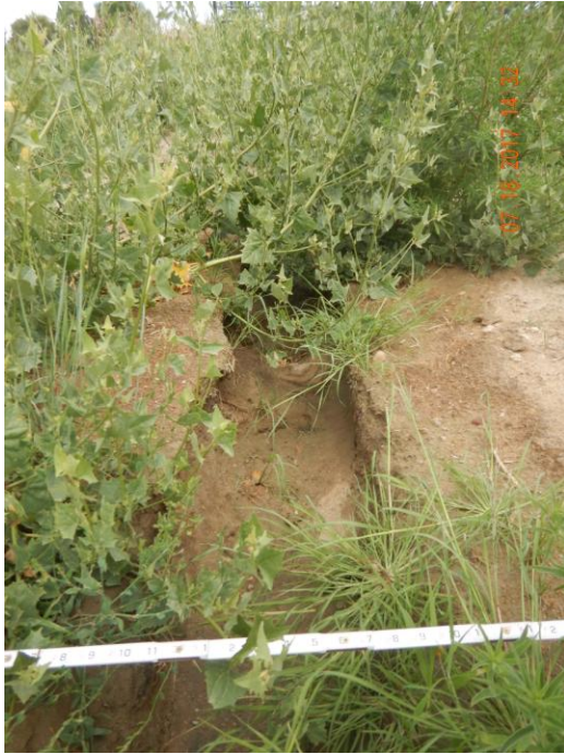
Photo 5: Photo taken from the north end of the location. Photo shows stormwater erosion occurring throughout the reclamation / remediation area. 6 foot measuring stick for reference. Location appears to have had a seeding attempted, however location was not seeding along the contour of the slope. This has facilitated erosion on the location.
