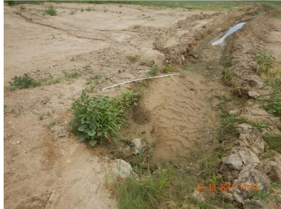
Photo 2: Photo taken from the southwest end of the location, facing southeast. Photo shows sediment laden stormwater runoff from the location has deposited into an irrigation ditch on the west end of the location. 6 foot measuring stick for reference.
