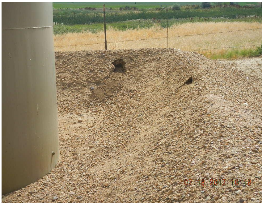
Photo 3 Compromised berm from west
