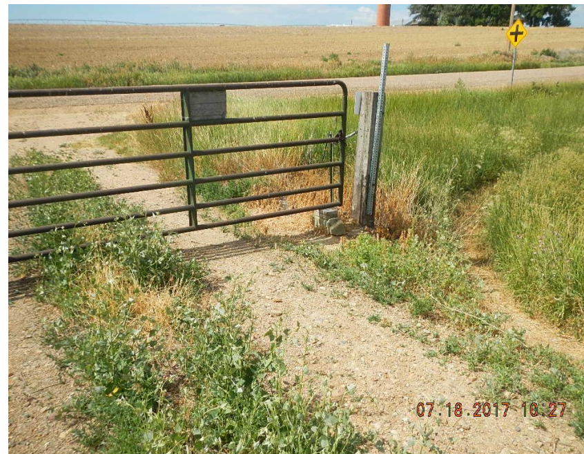
Photo 8 Gate requires maintenance note blocking under end of gate from north
