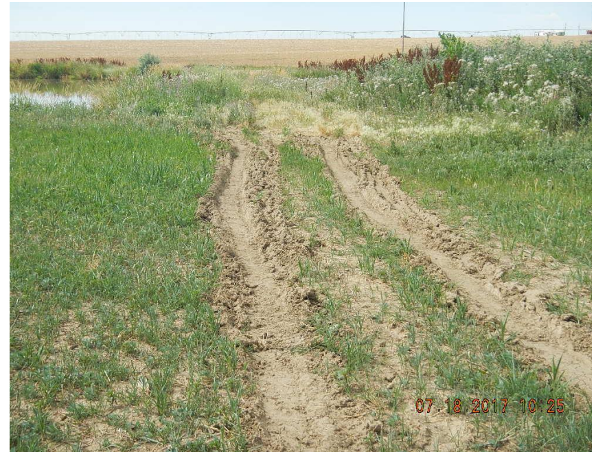
Photo 6 Rutting on access road from north
