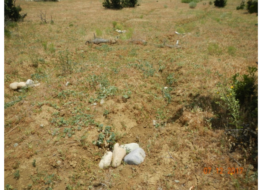
Photo 6: View of erosional channels that formed downstream of culvert shown in Photo 5. Cobble and wattle are not sufficient stormwater controls for this area. Permanent erosion controls need to be installed before the variance will be passed.
