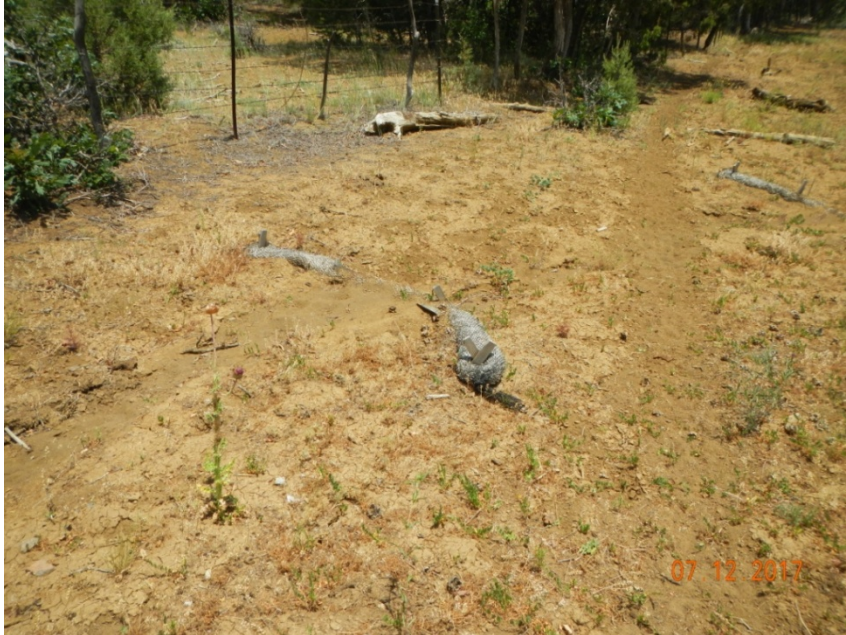
Photo 3: View of wattle that is no longer functioning within the northeastern corner of the project area. Permanent BMPs need to be installed to prevent erosion in this area.
