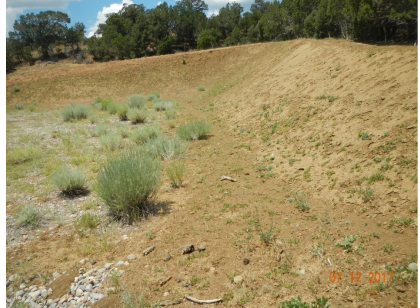
Photo 4: View of the northern and western cut-slopes from the northeastern corner facing westward. Exposed slopes need to be better stabilized with vegetation.
