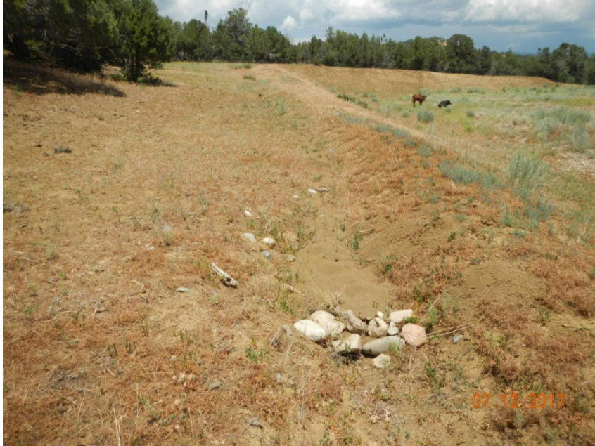
Photo 7: View of diversion channel in the western portion of the project area. Cobble check dam is full of sediment and will soon be eroding around the sides. This needs to be maintained, and expanded to provide longer term erosion control.
