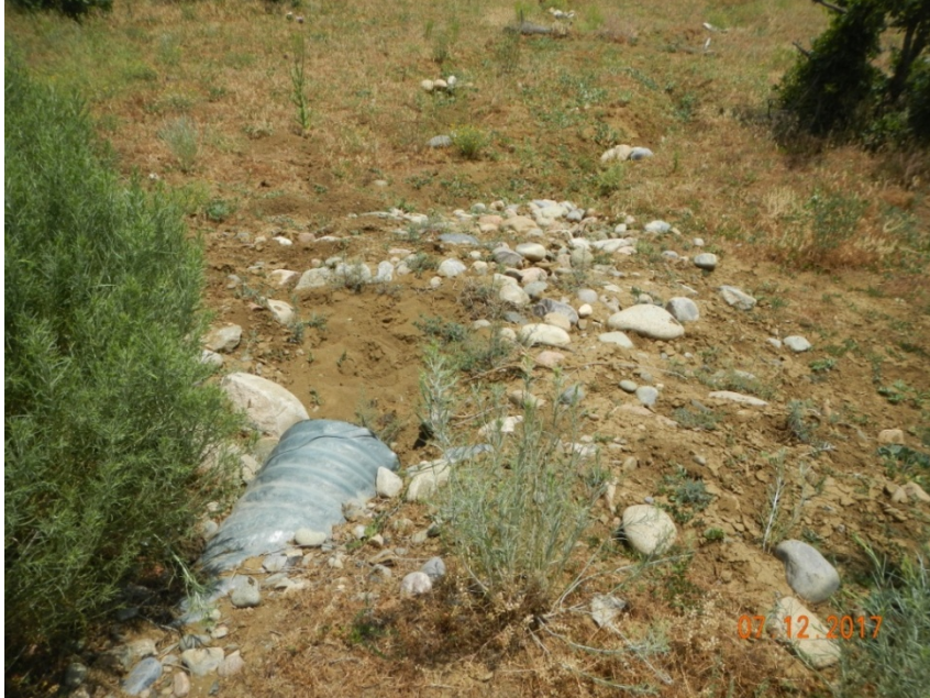
Photo 5: View of culvert outlet near the entrance to the well pad. Sediment is accumulating here and cobble BMP is not sufficient stormwater control for this area.
