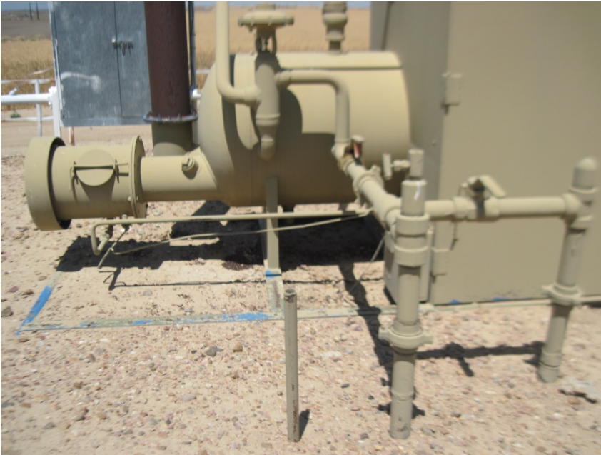
1" RISER IN NOT MARKED AT SEPERATOR
