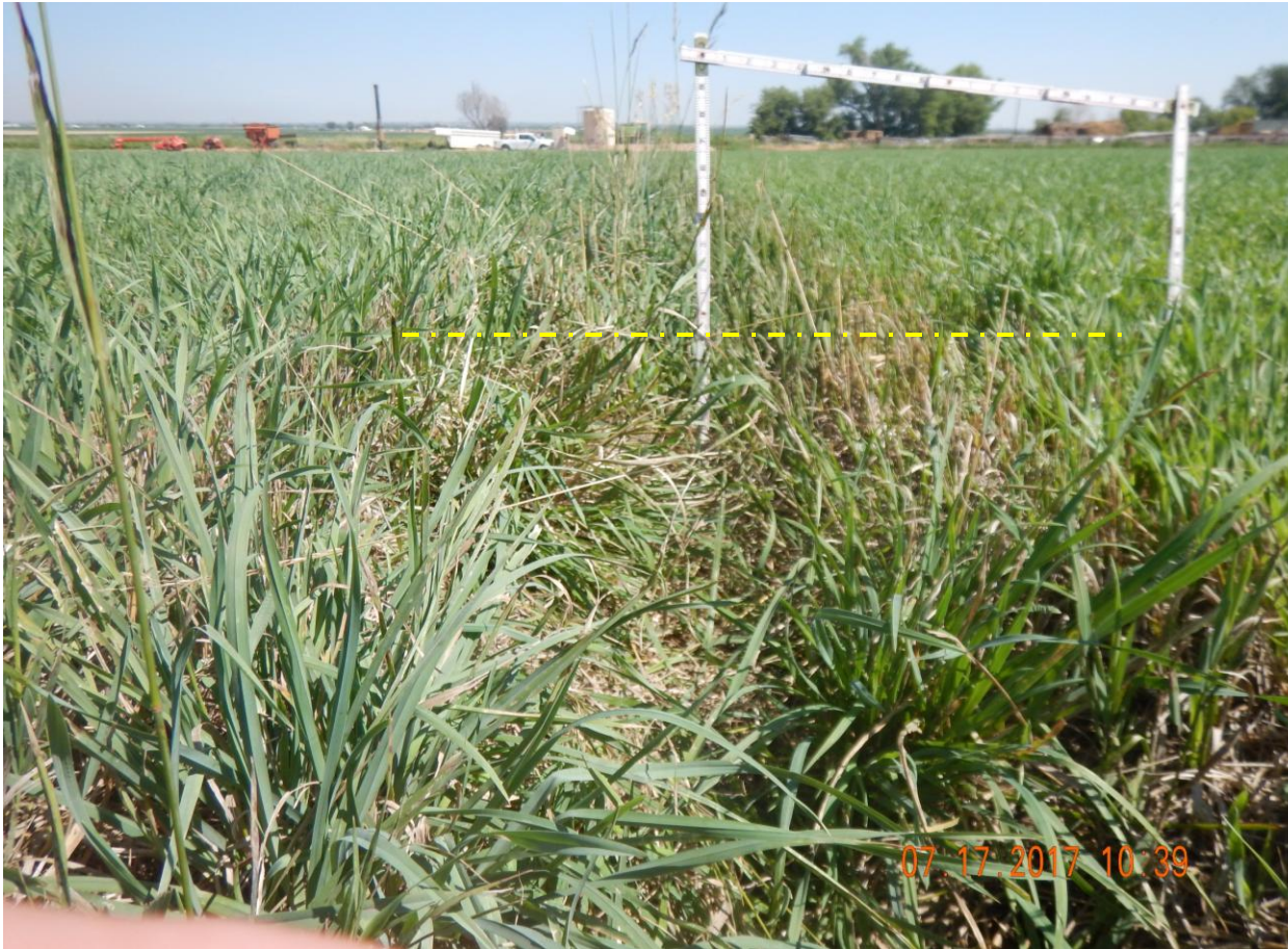
Photo 6: Photo taken from the access road. Photo shows rut in areas a foot deep (indicated by yellow line) or greater remain along access road. This indicates road has not been re-contoured or re-graded in accordance to COGCC 1000 series reclamation standards.
