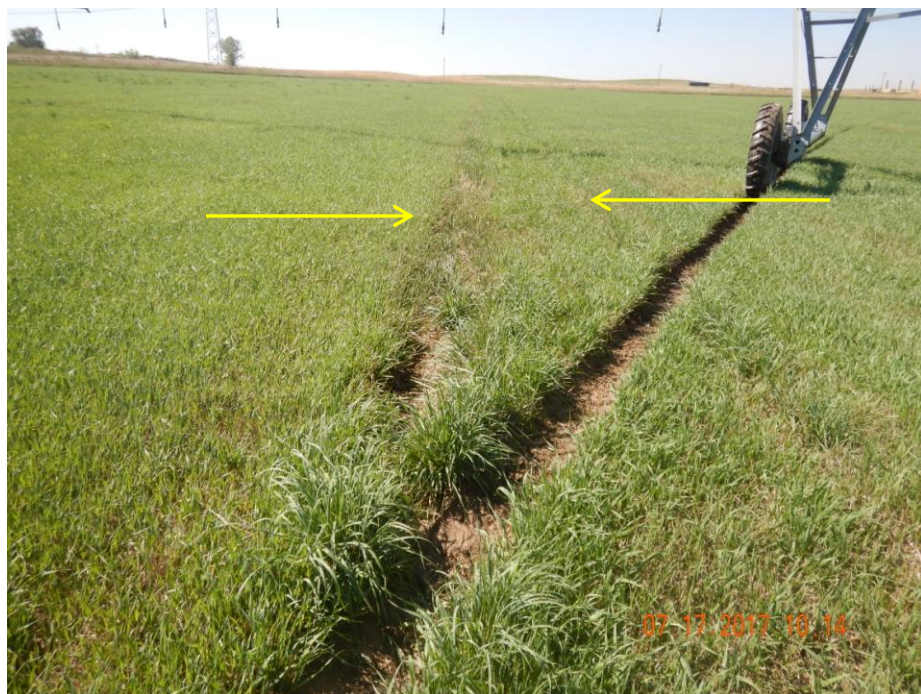
Photo 7: Photo taken from the access road, facing south. Photo shows ruts remain evident along access road (yellow arrows). It appears road had not been re-contoured or re-graded in accordance to COGCC 1000 series reclamation standards.
