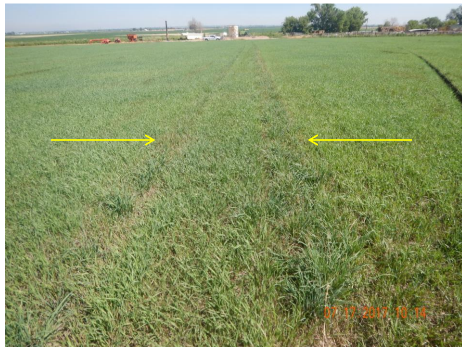
Photo 8: Photo taken from the access road, facing north. Photo shows ruts remain evident along access road (yellow arrows). It appears road had not been re-contoured or re-graded in accordance to COGCC 1000 series reclamation standards.
