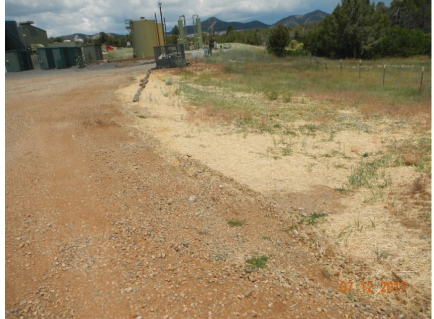
Photo 2: View of eastern portion of the project area showing mulched areas and wattles from the southeastern edge facing northward.
