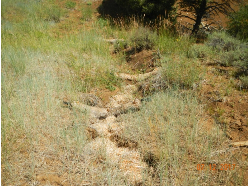
Photo 3: View of new stormwater controls installed in head-cut area at culvert outlet.
