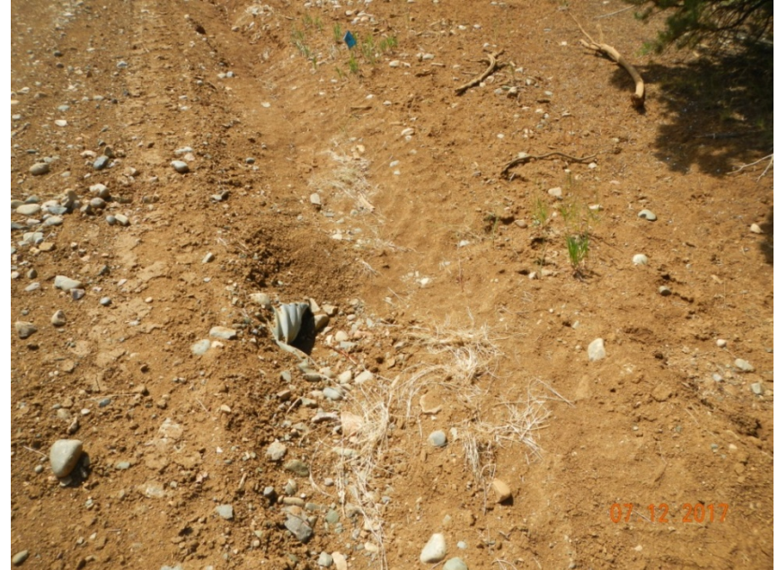
Photo 4: View of damaged culvert inlet at the well pad entrance.
