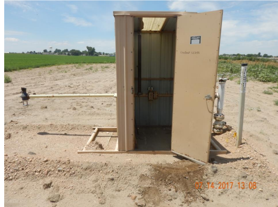
Photo 2: Photo of meter shed remaining at battery location. 1004.a reclamation rules require removal of all debris, abandoned gathering line risers, and flowline risers, and equipment within three months of plugging (12/09/2016) the associated facility. Meter shed needs to be removed and location reseeded .
