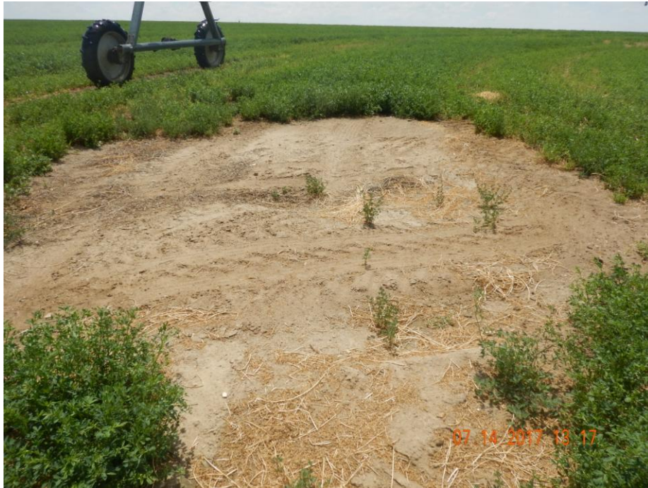
Photo 4: Photo taken from the well location. Photo shows subsidence occurring at well. Photo also shows that well does not appear to have been reseeded and area remains bare with no sign of germination or growth from the spring growing season.
