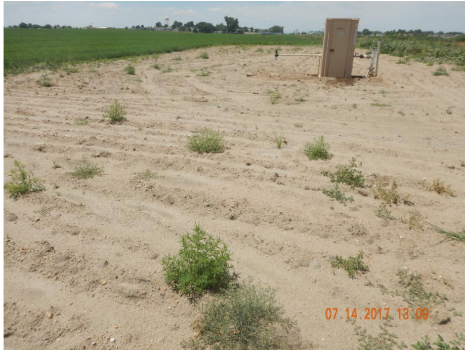
Photo 1: Photo taken from the east end of the battery location, facing west. Photo shows all facilities except meter shed has been removed. Location appears to have been cross-ripped. 1004.a reclamation rules require removal of all debris, abandoned gathering line risers, and flowline risers, and equipment within three months of plugging (12/09/2016) the associated facility. Meter shed needs to be removed and location reseeded .
