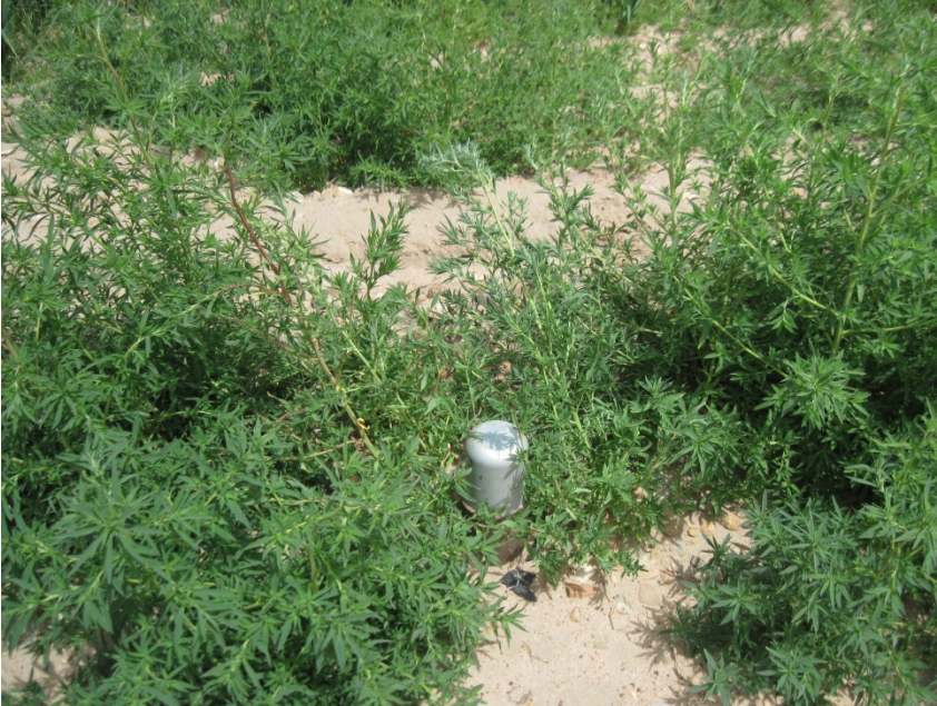
3" RISER NOT MARKED JAMES DAMIANA #2 SOUTH OF SEPERATOR
