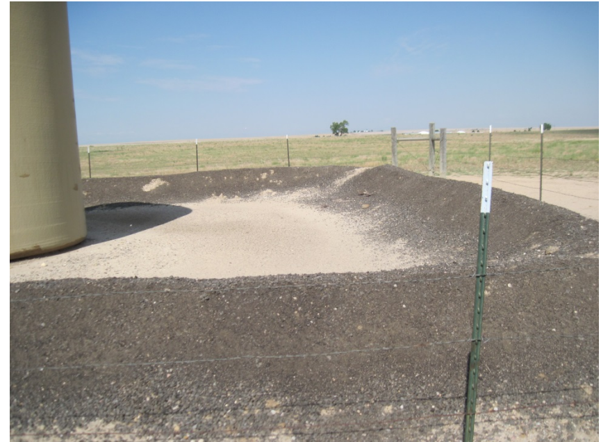
Berms repaired around tank battery
