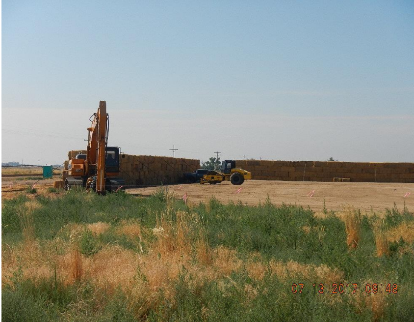
Photo 3 Sound mitigation bales on south and southeast corner of location.
