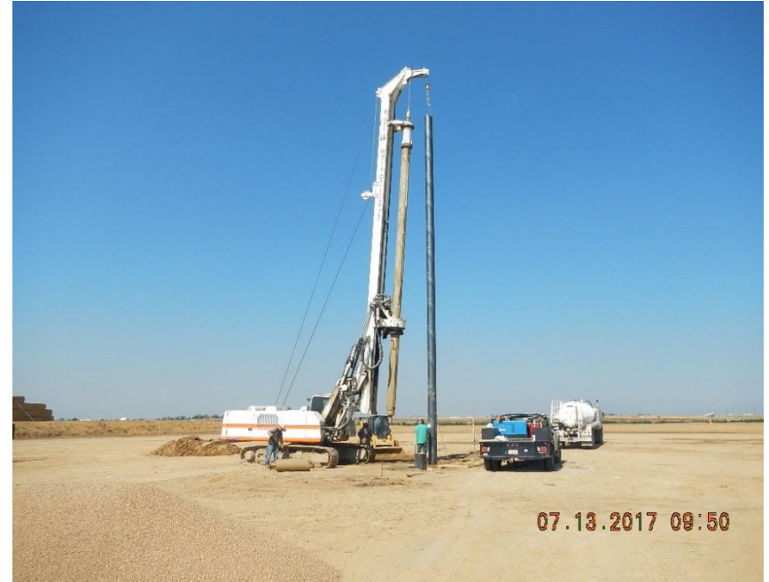
Photo 4 Pete Martin R-12 rig Welding of rat hole casing underway from east.
