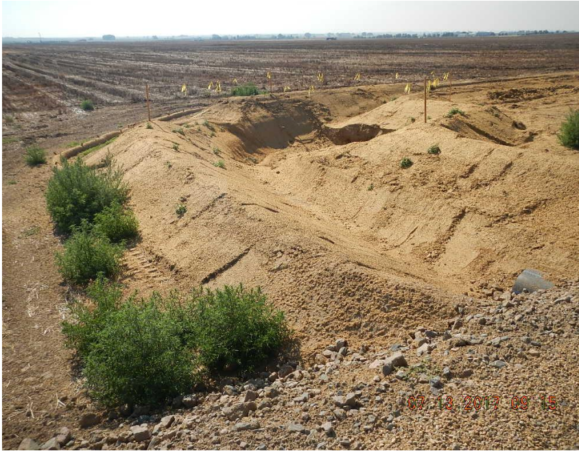
Photo 3 Storm water BMP's on northeast corner of location.
