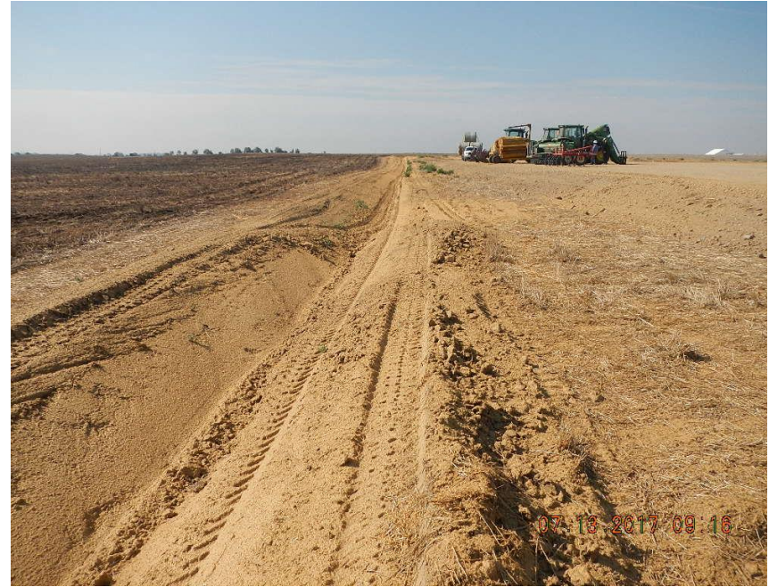
Photo 4 Ditch along east side of location from north
