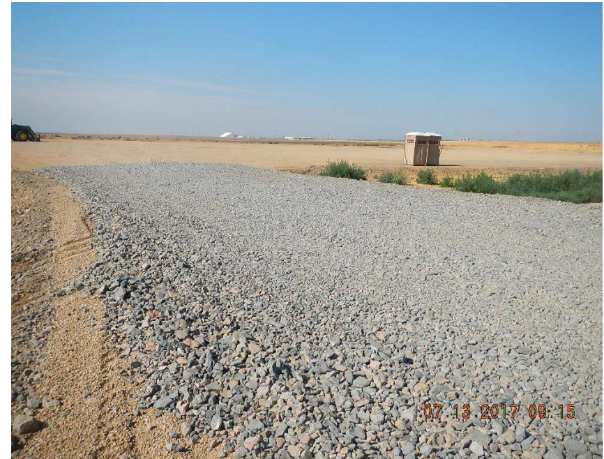
Photo 2 Entrance track pad from northeast
