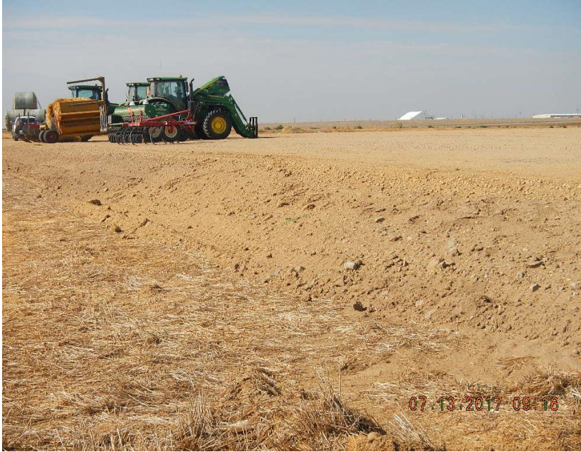
Photo 5 Cross section of fill from east approximate 4 ft thick
