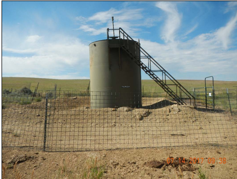
Photo 1. No contents, NFPA, or capacity on tank.
