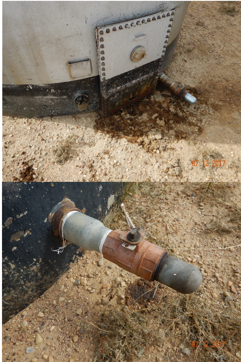
Figure 7 - Oil-stained soil (oily waste) beneath valves on north and south sides of crude oil AST.
