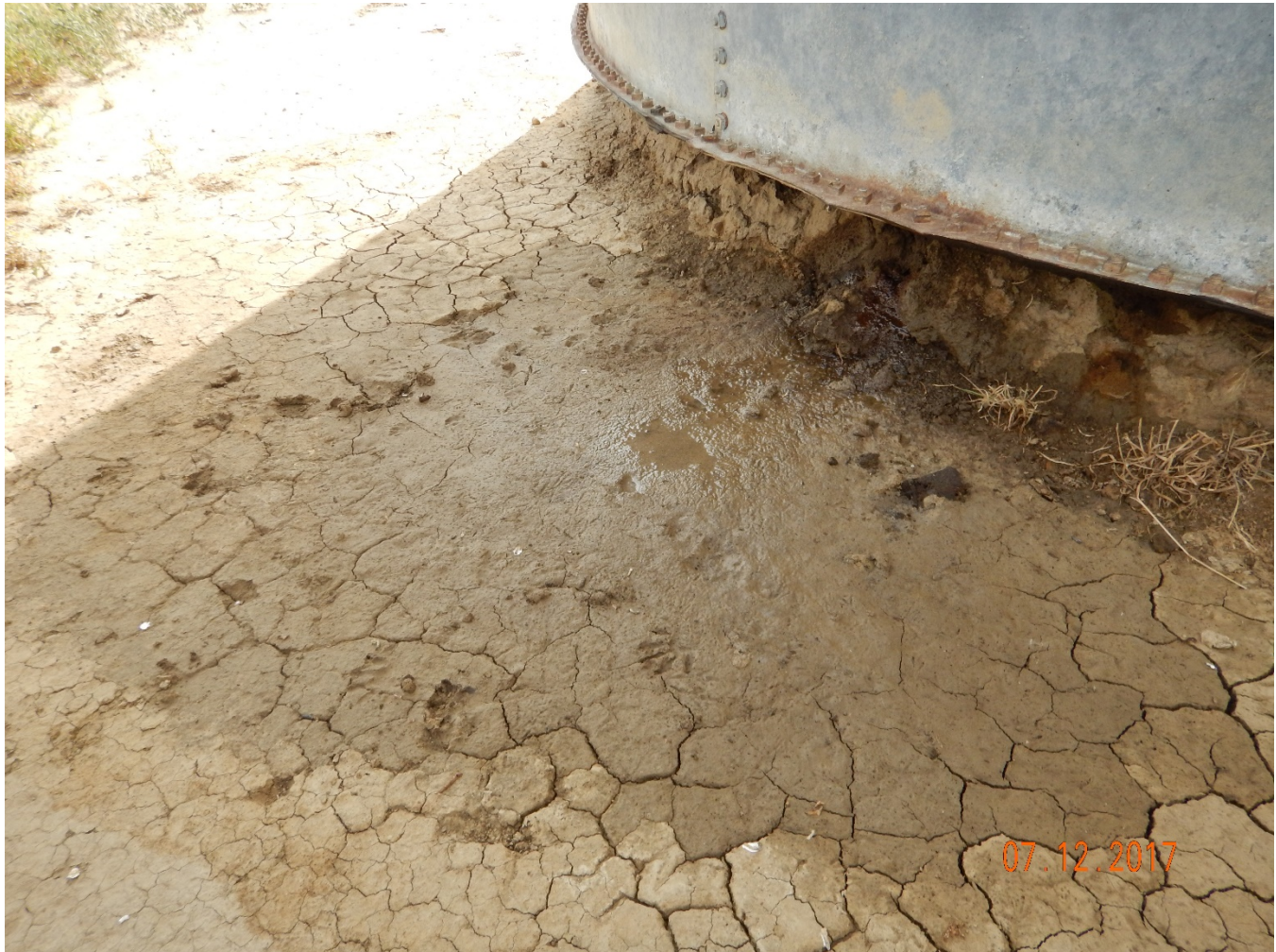
Figure 11 - Puddle was observed on north side of northern steel panel tank. Water was observed dripping from tank into puddle. A contractor on site was notified of this issue during the field inspection and a follow-up call was made to the operator the following day.
