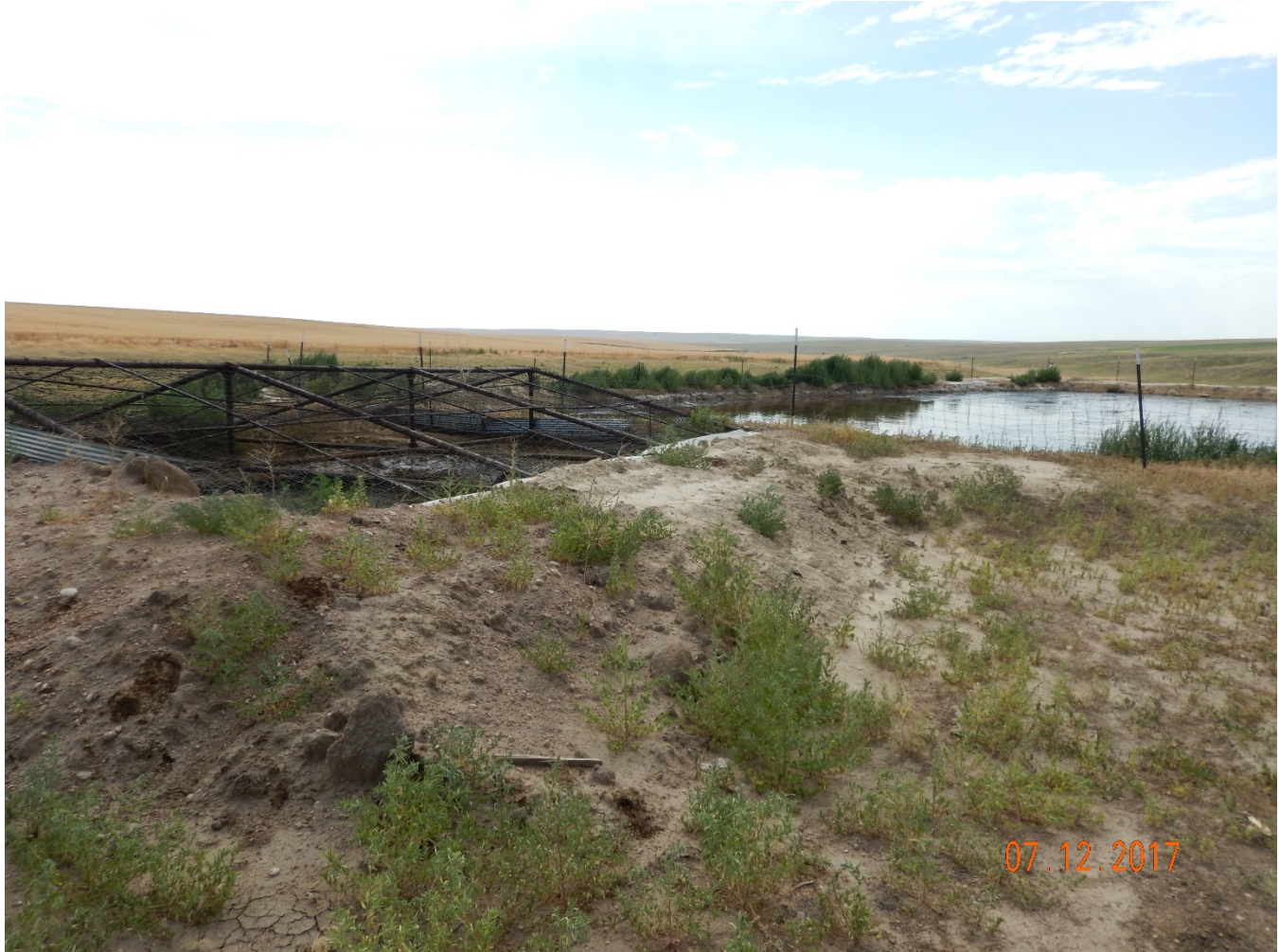
Figure 14 - Price-Degenhart 1 pit complex. Netted, unlined skim pit in foreground (left) with unlined produced water pit in background (right).
