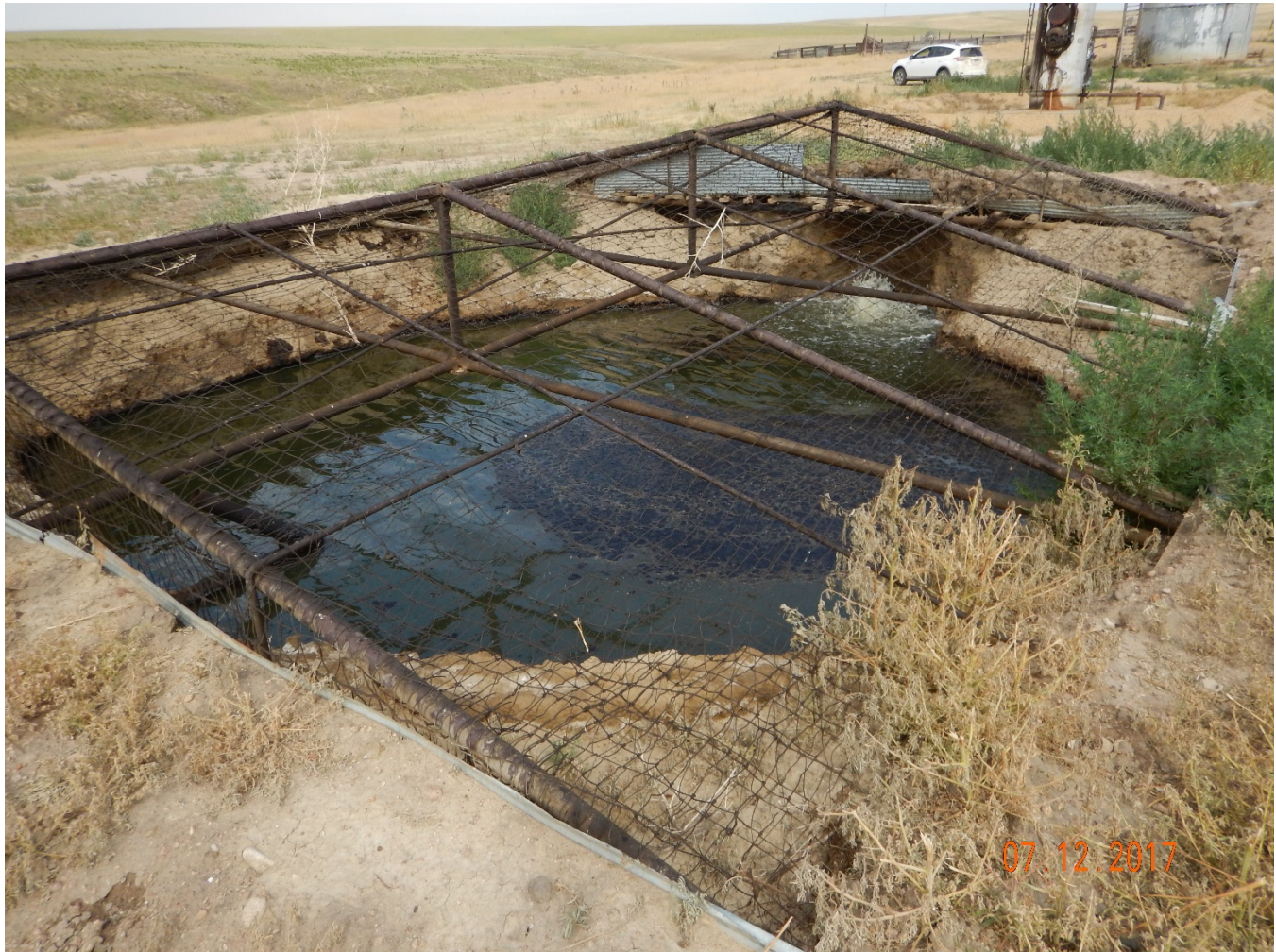
Figure 15 – View of unlined skim pit, COGCC Facility ID #104647, from SE corner. Note oil remaining on pit and berms. Continued operation of an unlined skim pit is a violation of Rule 904.a.(4), presence of oil on the pit is a violation of Rule 902.c and Rule 323.
