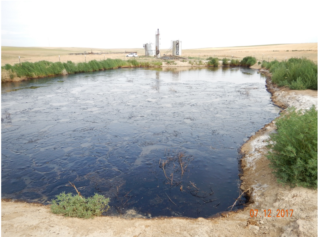
Figure 16 - View of unlined produced water pit, COGCC Facility ID #114378, from SE corner. Note: weeds growing into berms and continued presence of oil on pit, in violation of Rule 902.c and Rule 323.
