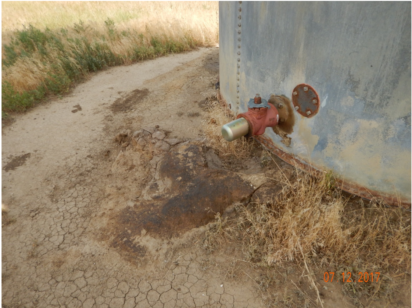
Figure 10 – Accumulation of oily waste beneath valve on west side of northern panel tank.
