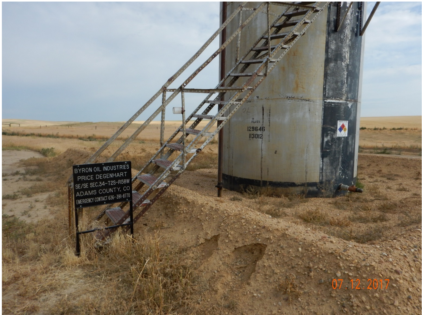
Figure 6 - Tank Battery sign and crude oil AST. Note: weeds have been addressed, but berm is eroded.
