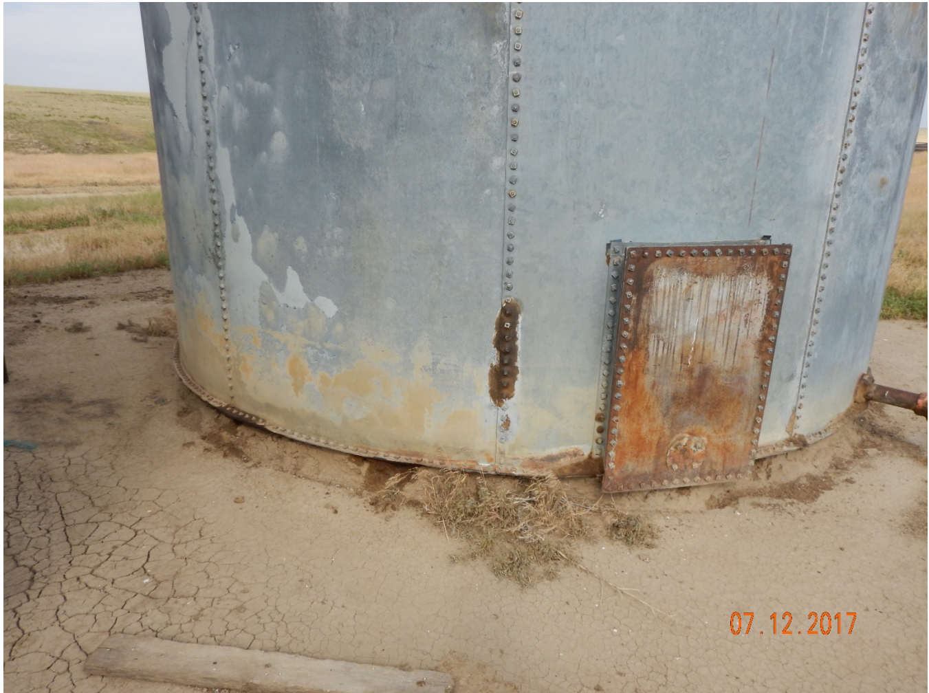
Figure 9 - Historical accumulation of oily waste beneath tanks and seeping from tank bolts. Tanks likely contain tank bottoms.
