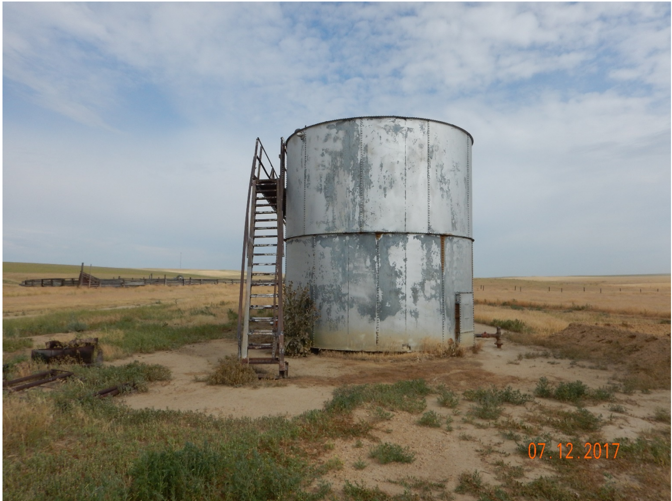
Figure 8 - View of unidentified, steel panel ASTs from the south. Operator confirmed that these tanks are inoperable and thereby subject to Rule 603.f for removal of unused equipment. Note asphaltic material (oily waste) immediately south of tank (in foreground) and tanks lack secondary containment.
