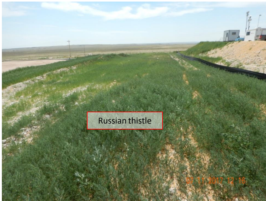
Photo 3. Photo taken between the Holliday pad and Tombstone pad on top of the topsoil stockpiles, facing South. Topsoil stockpile has predominately Russian thistle growth and Kochia growth which is not in compliance with Rule 1002.c. and Rule 1003. Hydromulch application was observed on the topsoil stockpile but is only a temporary BMP.
