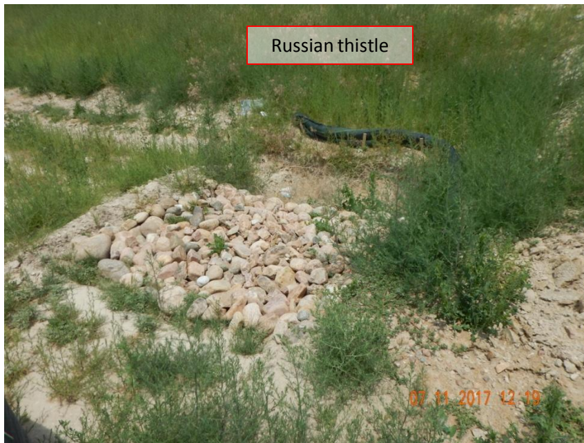
Photo 5. Photo taken from the southeastern Holliday pad, facing North. Sediment trap size was measured at ~5'x4'x1.5' (width x length x depth= 30ft 3 ) with a stabilized outlet.
