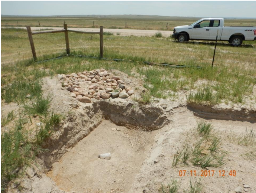
Photo 7. Photo taken from the southeast location of the Tombstone pad, facing South. Sediment trap size was measured at \sim 7' \times 4.5' \times 2' (width x length x depth= 63ft 3 ) with a stabilized outlet. Sediment discharge was observed beyond the outlet area and beyond the filtrex BMP along the corner of the fence. Refer to photos 9 & 10.
