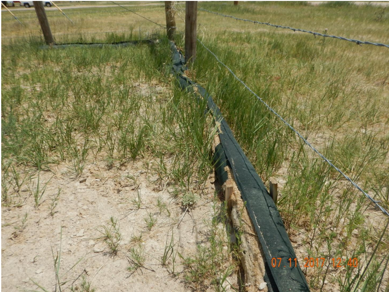
Photo 9. Close up photo taken just beyond the sediment trap at the corner of the fence, illustrating stormwater runoff appears to be washing hydromulch material and sediment off location over the filtrex BMP.
