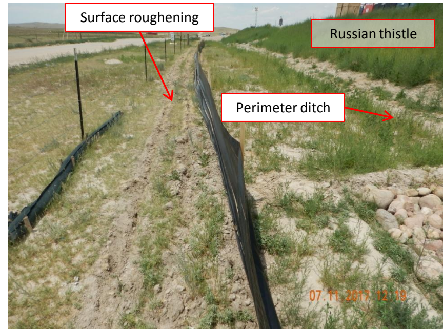
Photo 6. Photo taken from the southeastern Holliday pad, facing West. Silt fence improperly installed outside of the perimeter ditch, then surface roughening with filterxx BMP along a portion of the southeastern perimeter. Silt fence is only pinned down and not buried/back-filled/compacted. Also, silt fence stakes should be installed to the outside of the silt fence, not inside of the silt fence.
