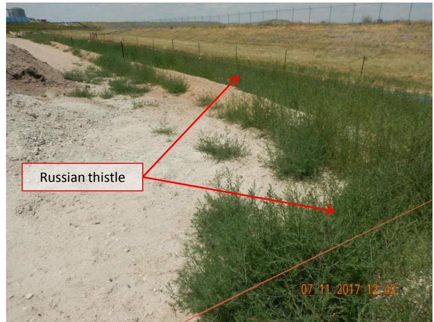
Photo 12. Photo taken from the northeast location of the Tombstone pad, facing Northwest. A berm ~18" has been constructed along the north, east and south pad perimeter, but does not appear to be properly compacted.
