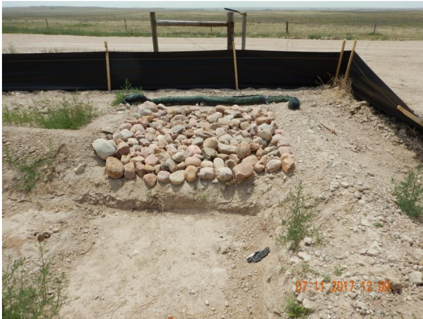
Photo 1. Photo taken from the southwest Holliday pad, facing South. Sediment trap size was measured at ~5'x4'x1.5' (width x length x depth= 30ft 3 ) with a stabilized outlet. Silt fence BMP has not been properly installed. Silt fence is only pinned down and not buried/back-filled/compacted. Also, silt fence stakes should be installed to the outside of the silt fence, not inside of the silt fence.
