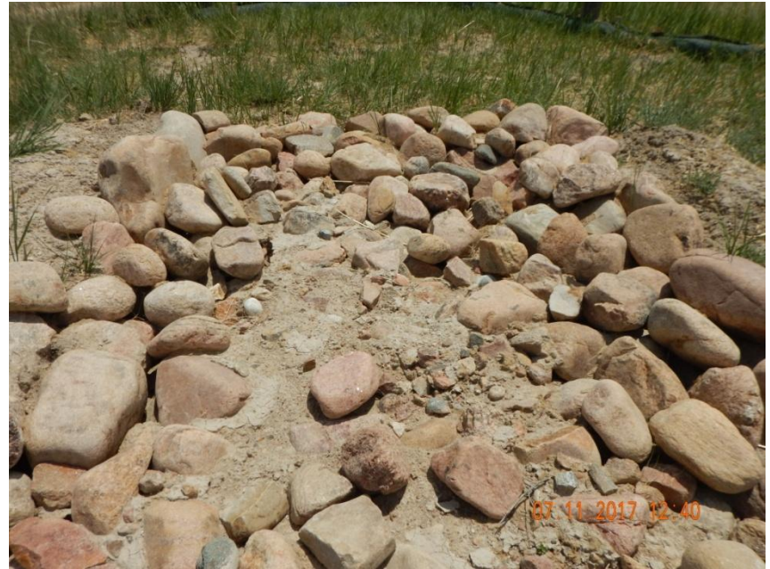
Photo 8. Close up photo taken from the outlet area of the sediment trap illustrating sediment build up which indicate the sediment trap is not built to a sufficient size.
