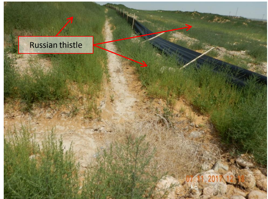
Photo 4. Photo taken from the southeast Holliday pad, facing North. Sediment trap size was measured at ~5'x4'x1.5' (width x length x depth= 30ft 3 ) with a stabilized outlet.. Silt fence has not been properly installed. Silt fence is only pinned down and not buried/back-filled/compacted. Also, silt fence stakes should be installed to the outside of the silt fence, not inside of the silt fence. Russian thistle growth observed throughout most disturbance areas.
